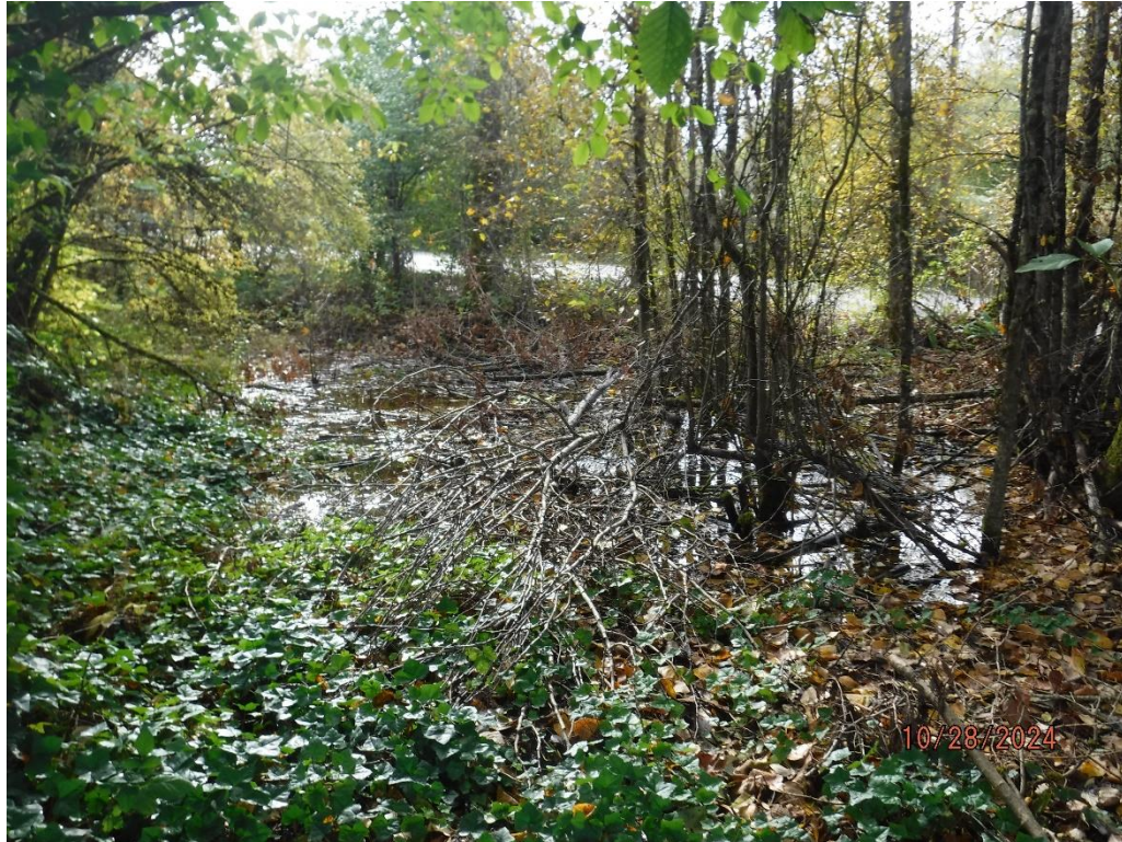
View of the northwestern corner of the project site (near SP8) during a period of seasonal rainfall. This area created topographic swale receives stormwater runoff from the school facilities and Fruitland Avenue prior to entering a culvert near the center right part of the photo. This swale appears to drain moderately well following seasonal storm events.
