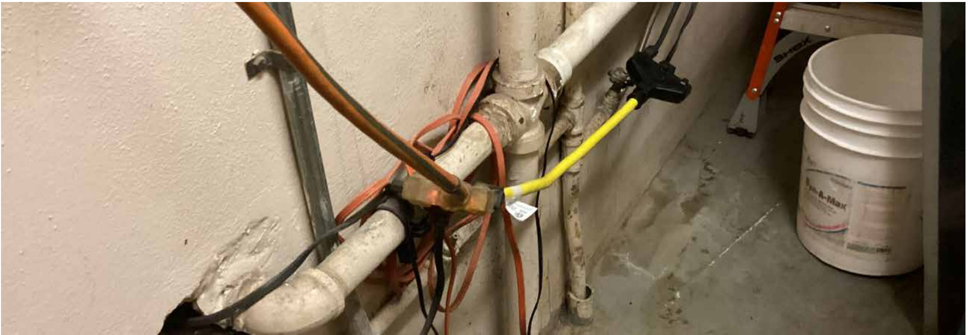
Extension Cord Used as Permanent Wiring
