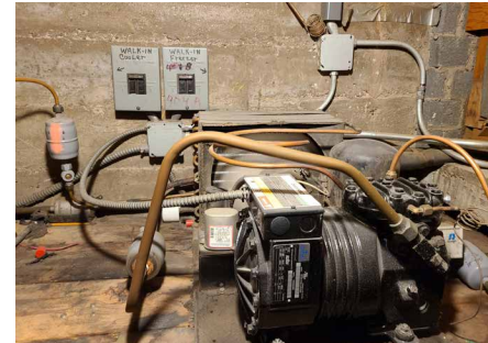
Walk-In Freezer + Cooler/Kitchen Compressor
