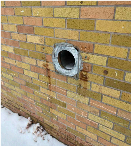
Missing Vent Cover/West Facade Near Door 23
