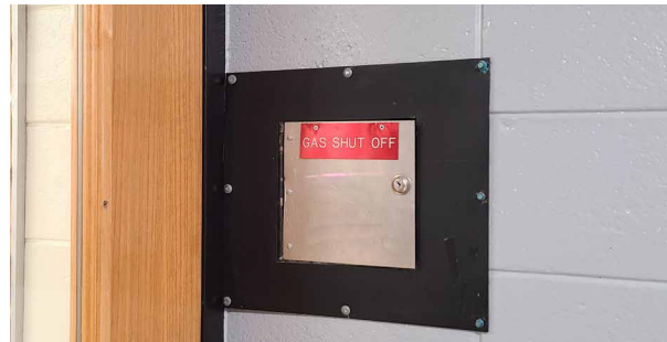
Emergency Gas Shut Off Valve 24/Science
