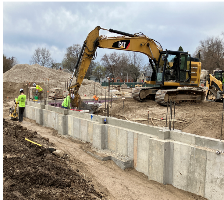
Foundation Walls & Column Piers
