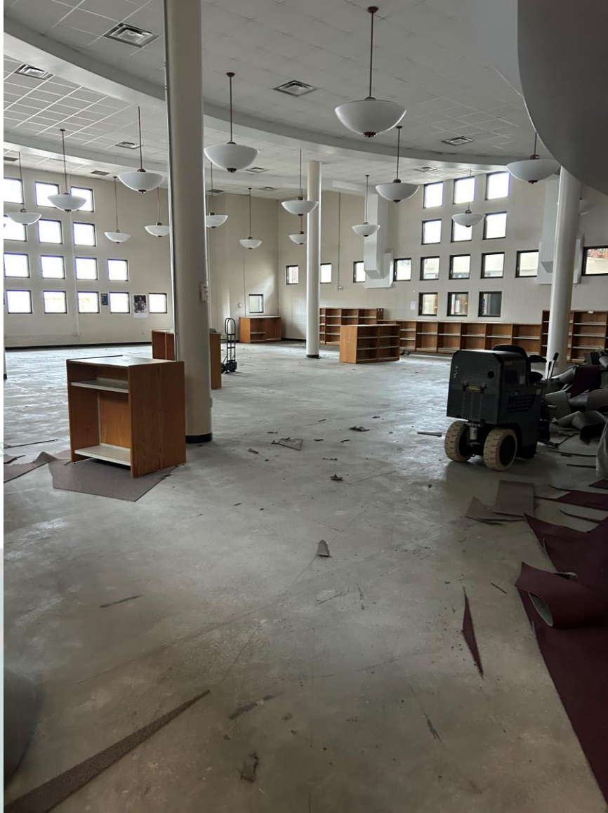
Carpet Removal and Flooring Work in Media Center
