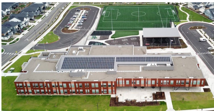
Tamarack Solar Panels
