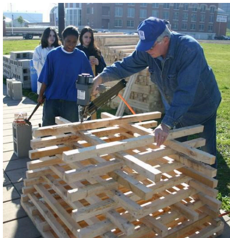
Figure 2. Photo Examples of Pennsylvania Porcupine Crib Construction
