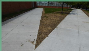
NEW SITE CONDITIONS
