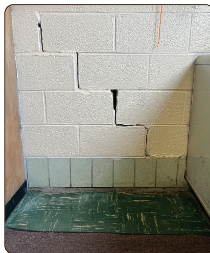
Over time, shifting and settling have caused cracks to form in the walls.
