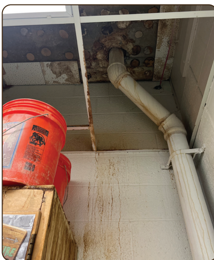
Aging pipes and ceiling leaks have caused significant water damage throughout the building.
