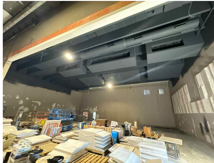
SVMS - Ceiling Dryfall & Walls Primed
