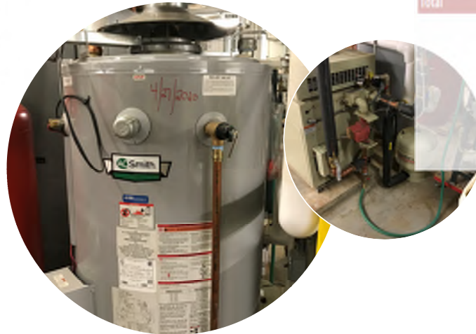
Water Heater & Expansion Tank Replacements
