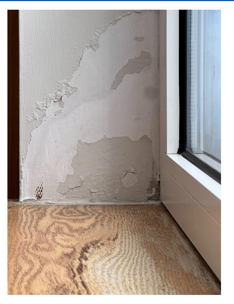
Rainwater is penetrating around some windows, impacting drywall and sills
