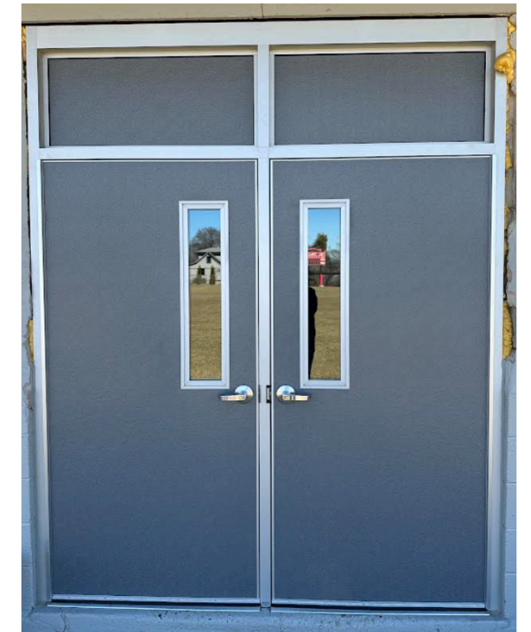
New Warming House Doors
