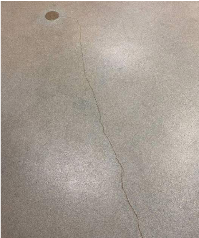
View of the crack in floor finishes on slab on grade.
