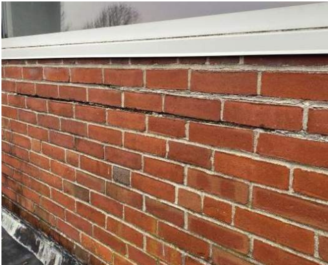
View of the cracks and signs of past repairs in exterior masonry façade.
