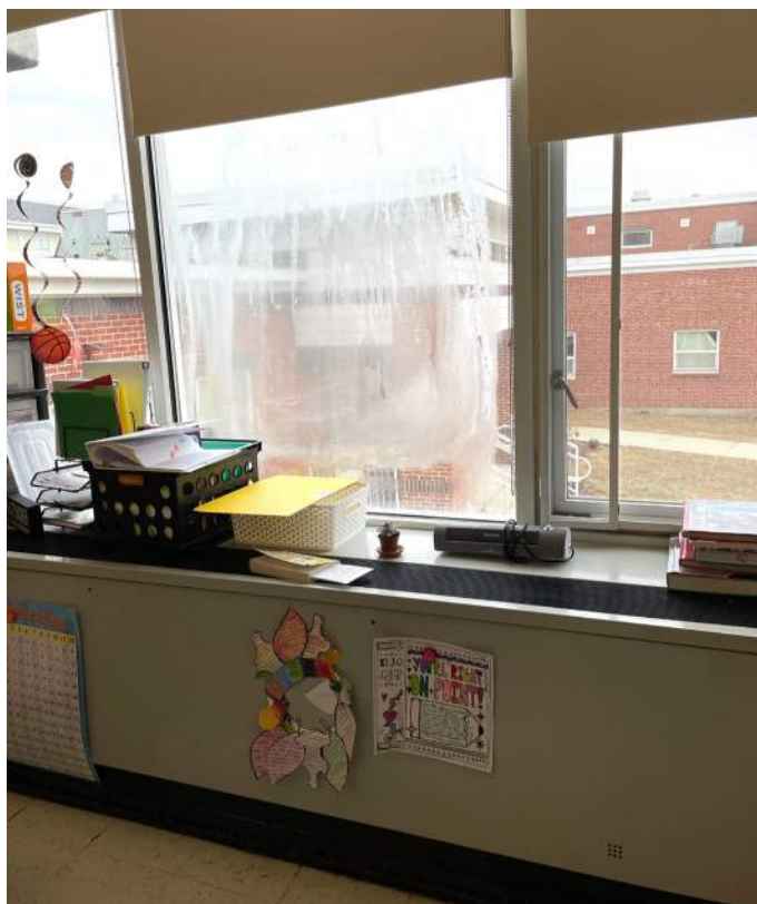
Condensation on window with broken seal above a typical classroom unit ventilator
