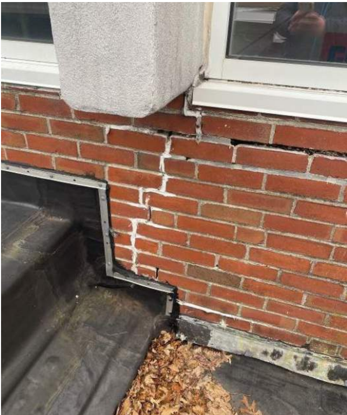
View of the cracks and signs of past repairs in exterior masonry façade.
