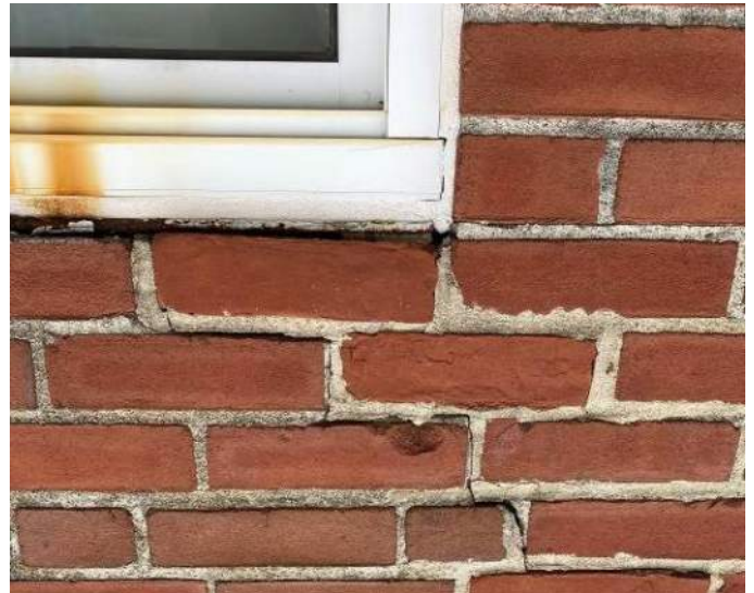
View of the rusted lintels and related cracks in the masonry.
