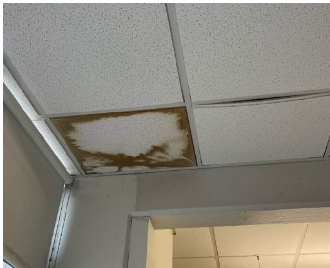
Untraced leak leading to growth on acoustic ceiling tile
