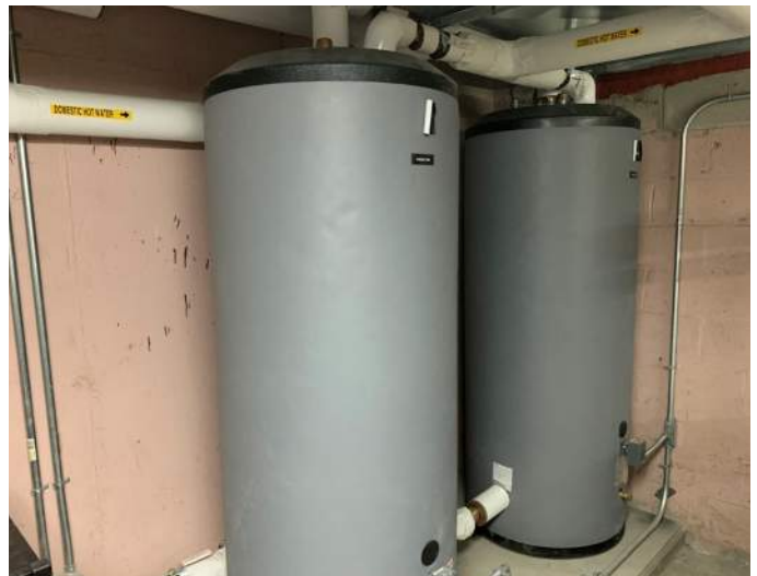
Duplex hot water tanks.
