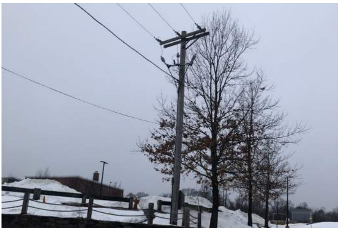
Electric Utility Co. Riser Pole.
