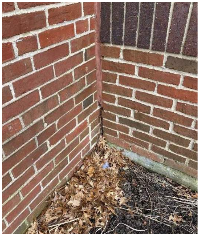
View of failed caulking in masonry control joints.
