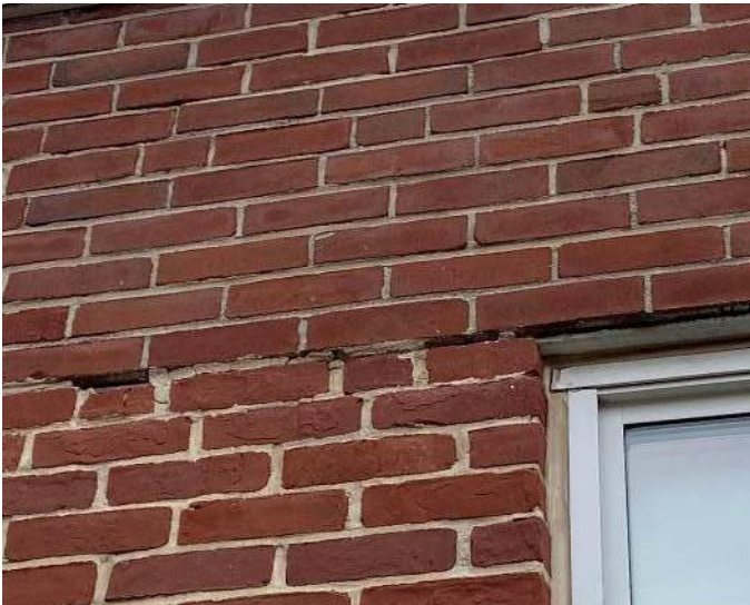
View of the rusted lintels and related cracks in the masonry.
