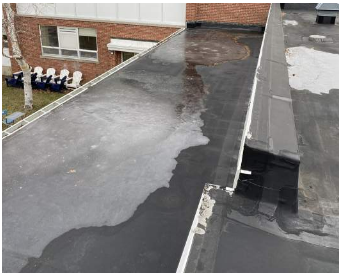
Typical EPDM roof ponding & tearing
