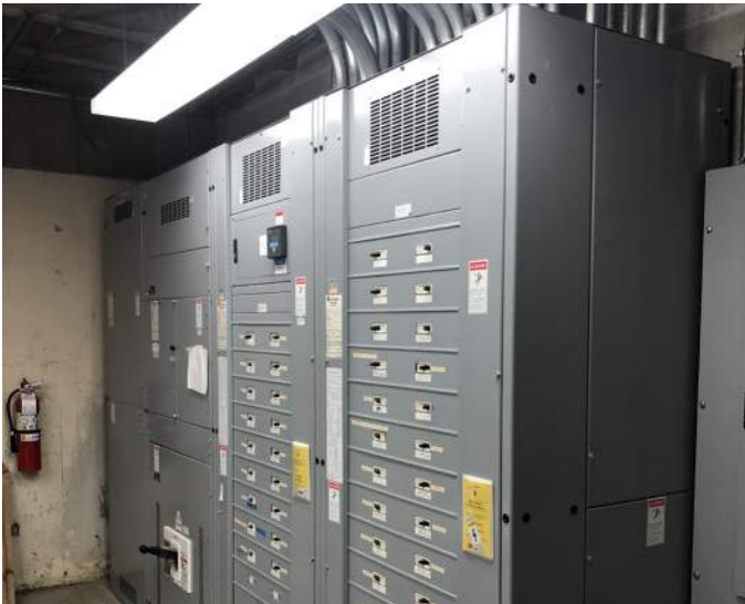
Switchboard and power distribution in main electric room.
