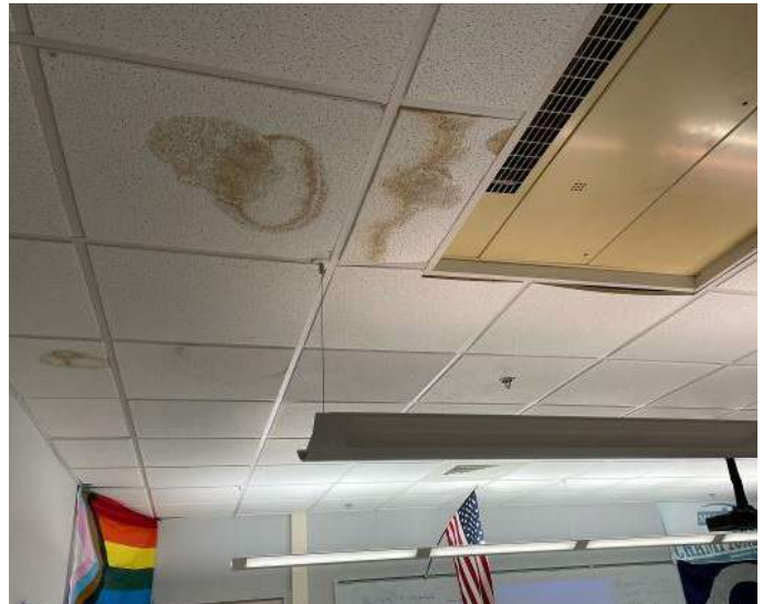
View of water stains in the ceiling.
