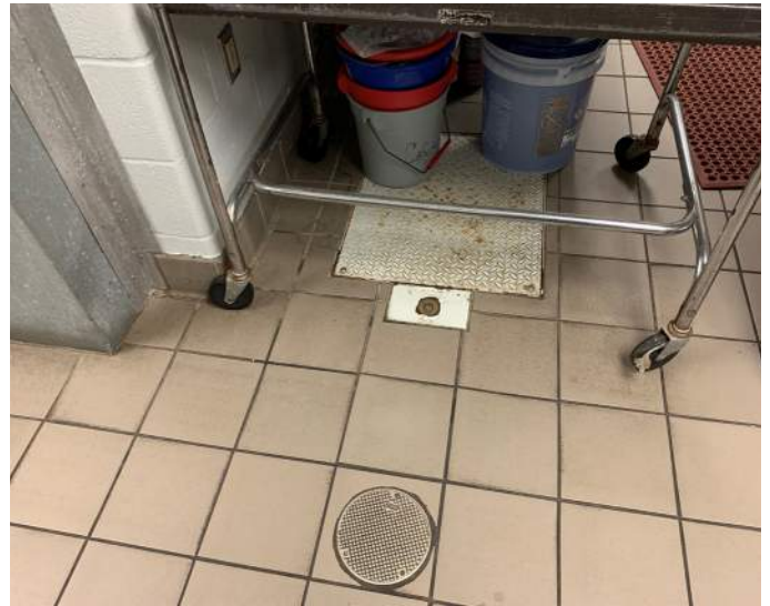
Recessed grease trap in kitchen.
