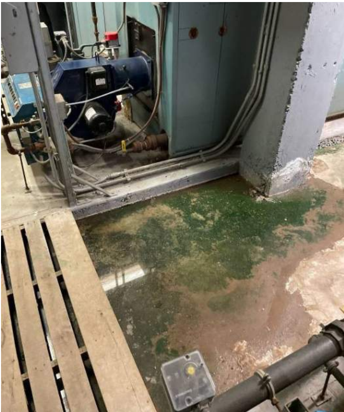
View of standing water in the mechanical room.
