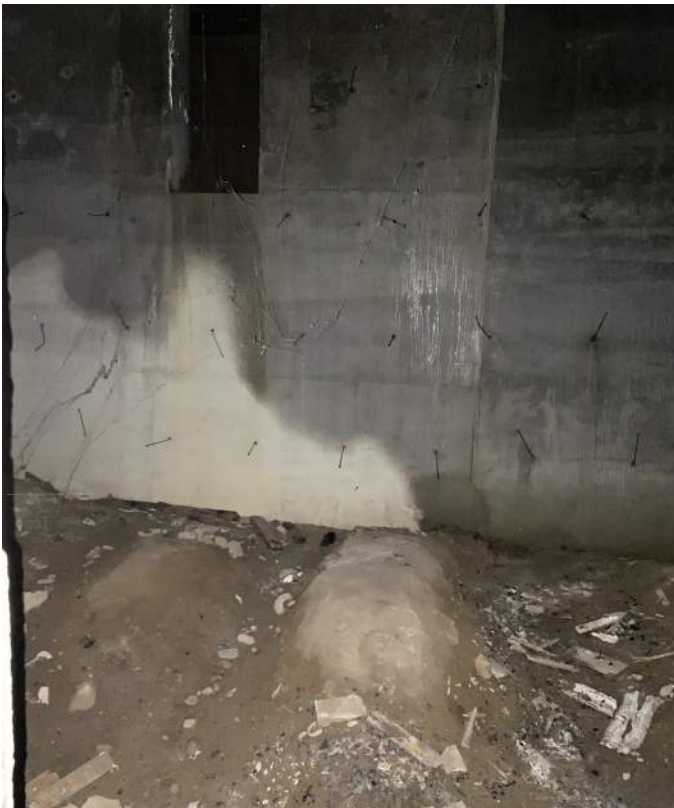
No insulation or waterproofing on face of foundation wall
