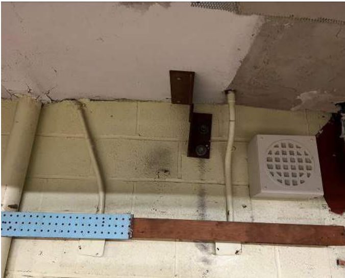
View of the seismic clips at top of the masonry walls.
