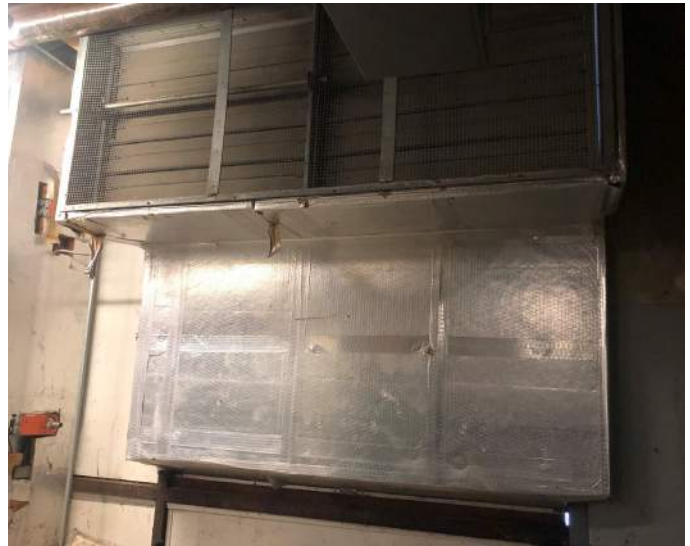
Combustion air intake.
