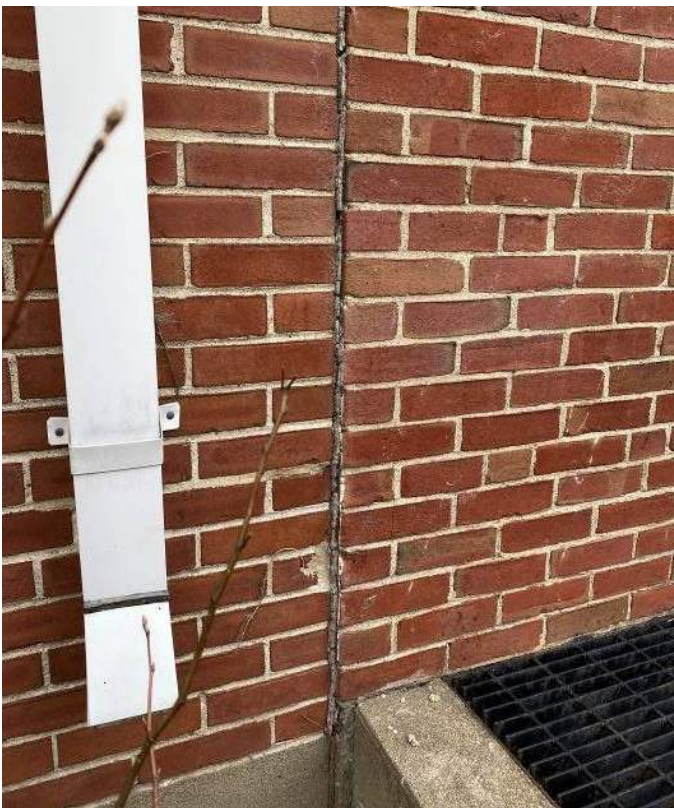
View of failed caulking in masonry control joints.
