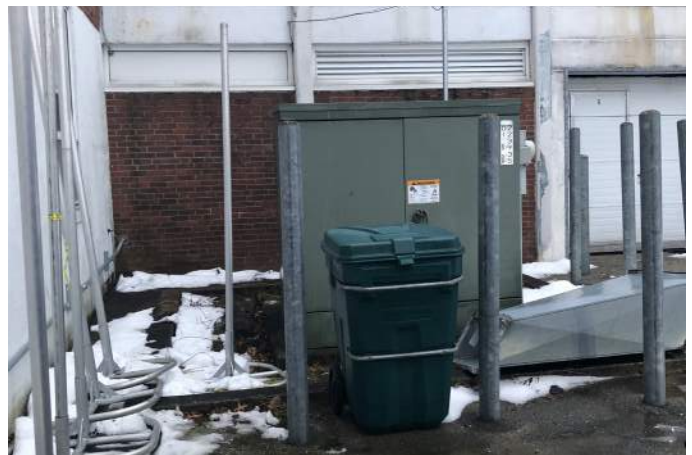
Electric Utility Co. Pad Mounted Transformer.
