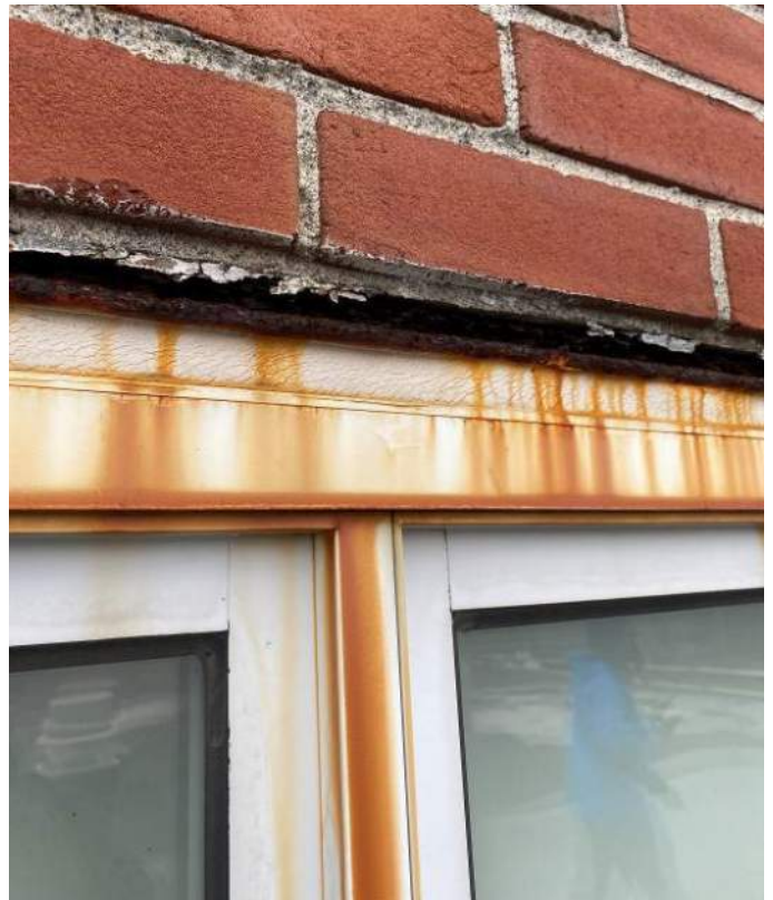
View of the rusted lintels and related cracks in the masonry.
