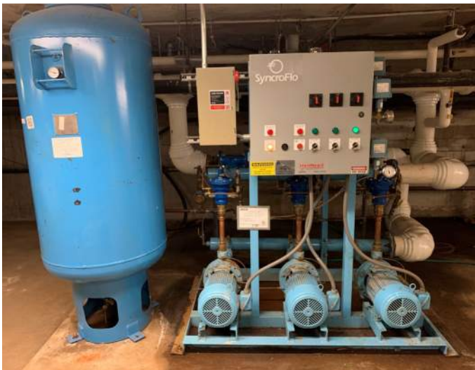
Triplex water booster pump.
