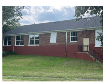
Field House Phase I is complete! Our Bulldogs will have access to it this Fall. Phase II starts next spring!
