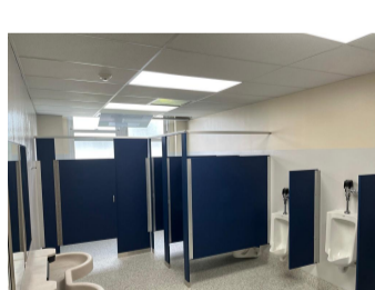
New bathrooms at JDHS and FMG are looking great!
