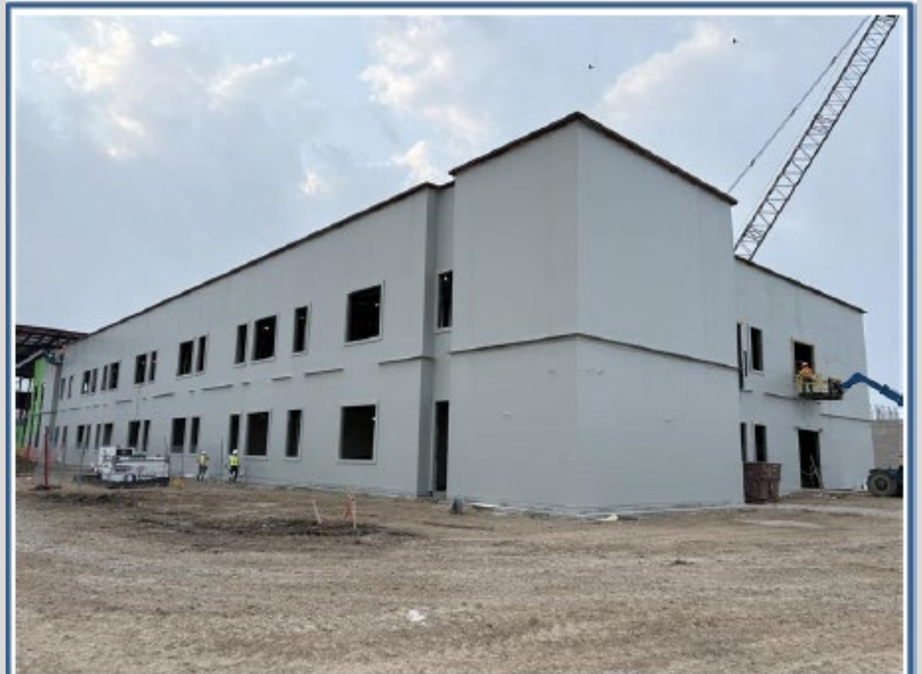
Area A Exterior Waterproofing
