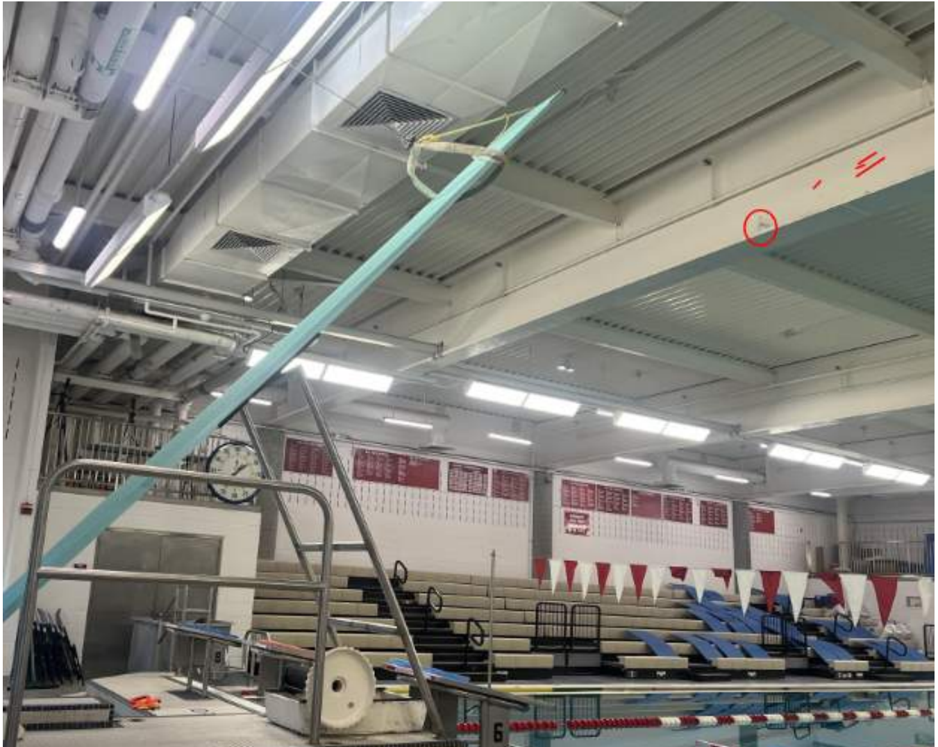
Photo 9: The steel girder, beams, ductwork and sprinkler piping are all within the required overhead clearance for diving, as shown in Figure 3.
