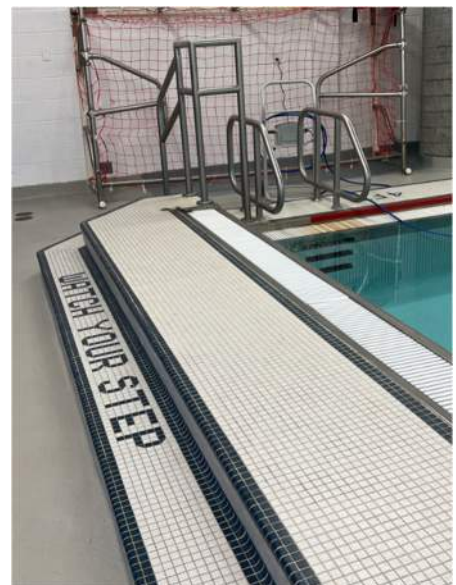
Photo 1 (Above): Overall view of pool from shallow-end. Pool edge is built up with a bulkhead curb and steps to form a recessed gutter on the touch walls.
