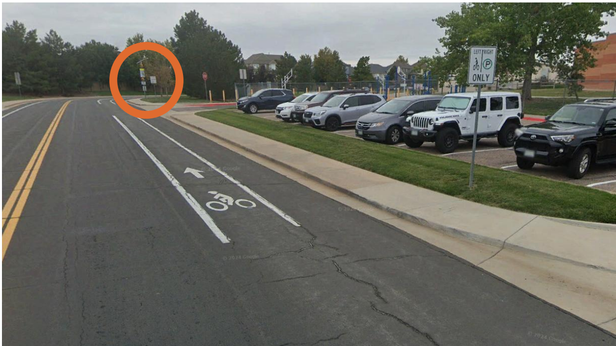
Figure 5 – Southbound School Zone Indicator
