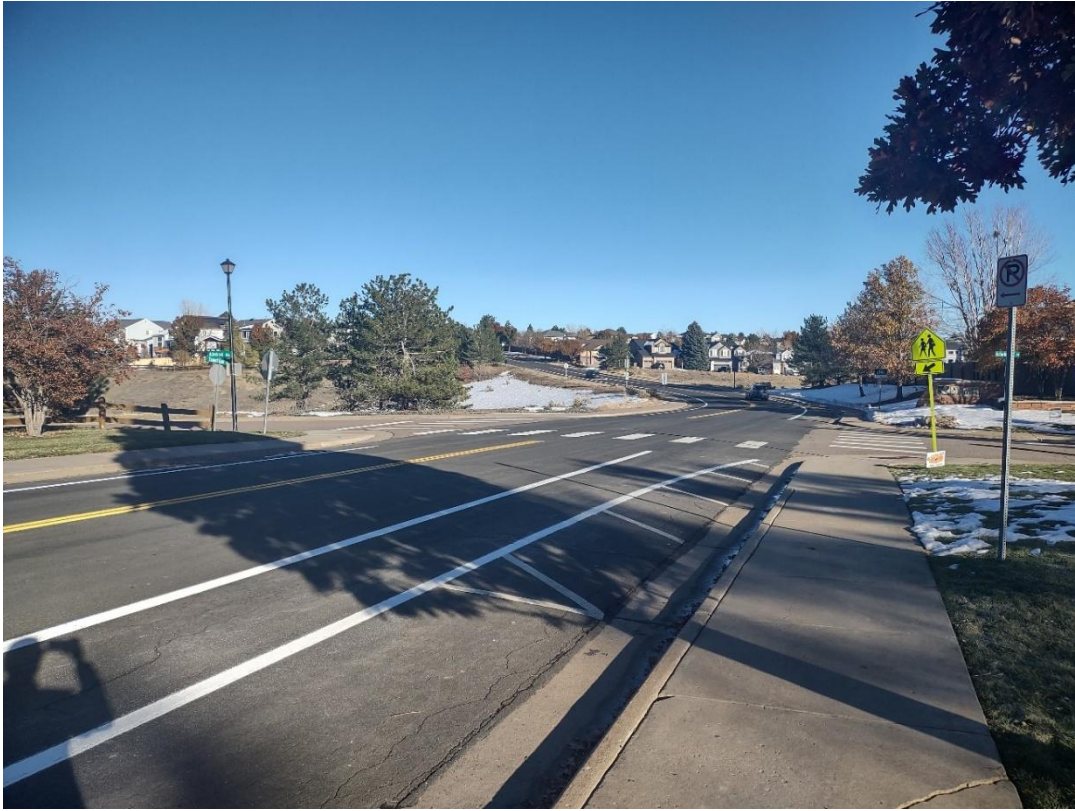
Figure 5 – No Parking Sign With Pavement Markings
