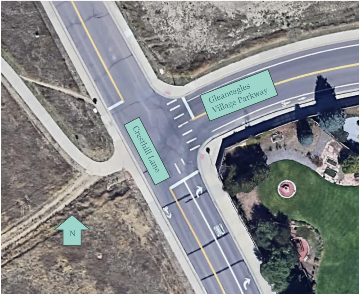
Figure 4 – Cresthill Lane at Gleaneagles Village Parkway
