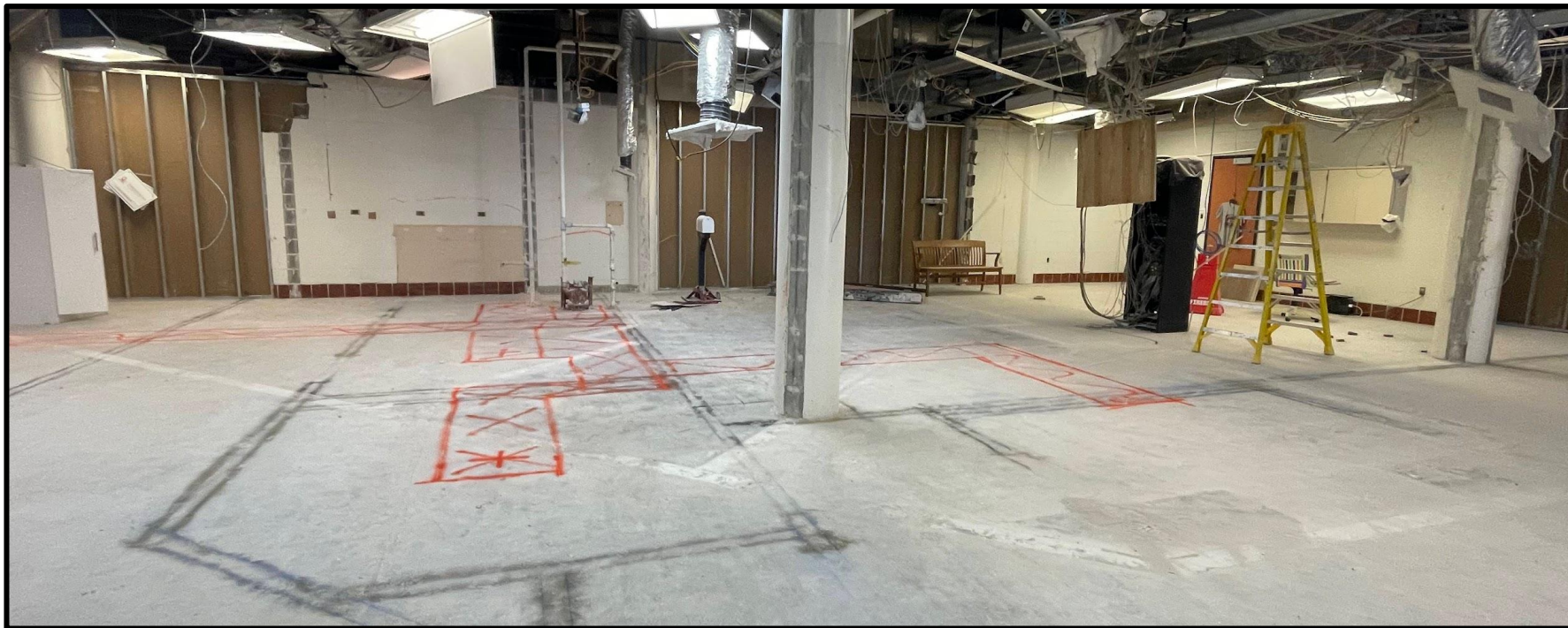
Roberts Road Elem. Demolition
