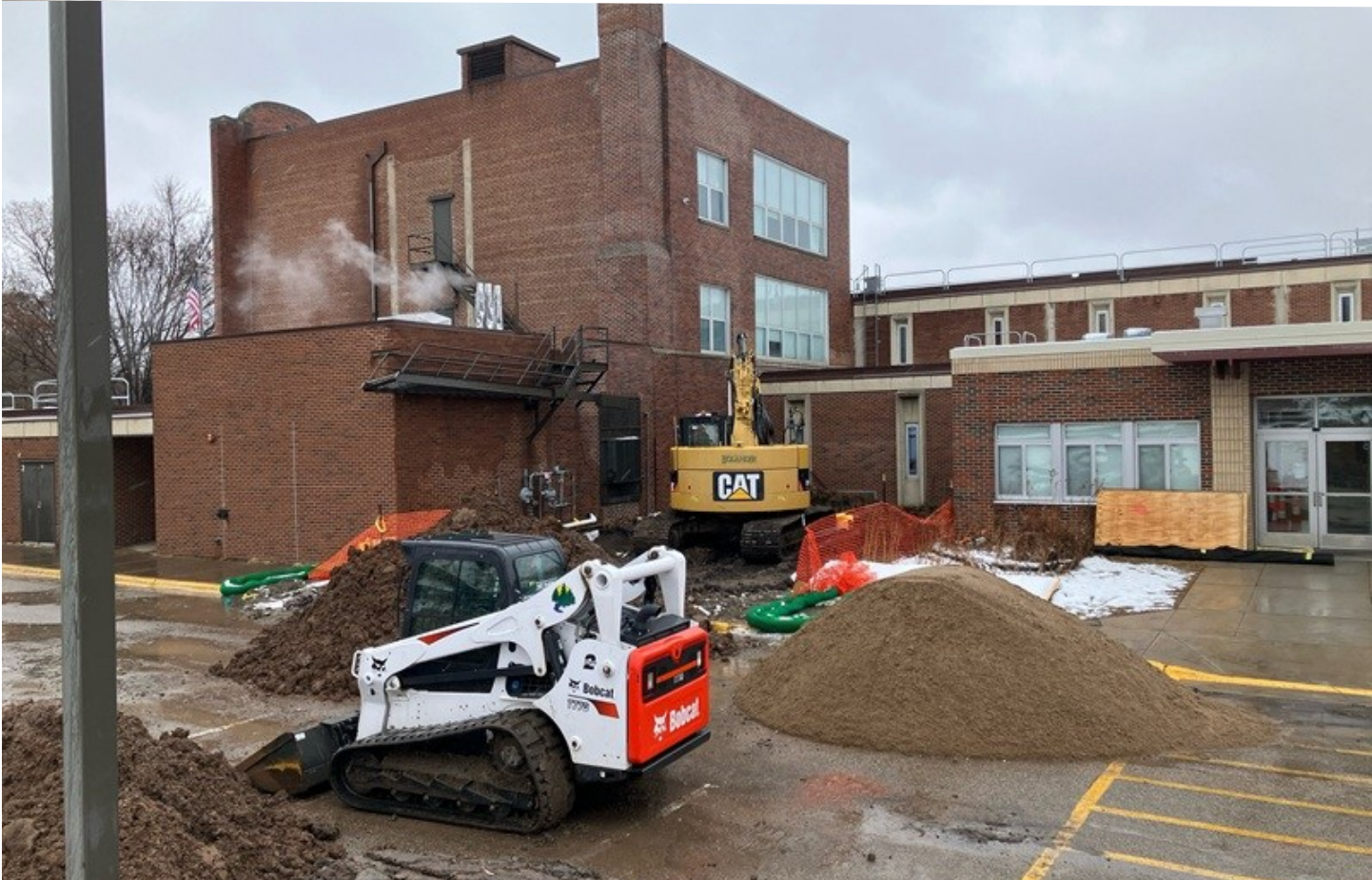
Storage tank removal (April 2025)
