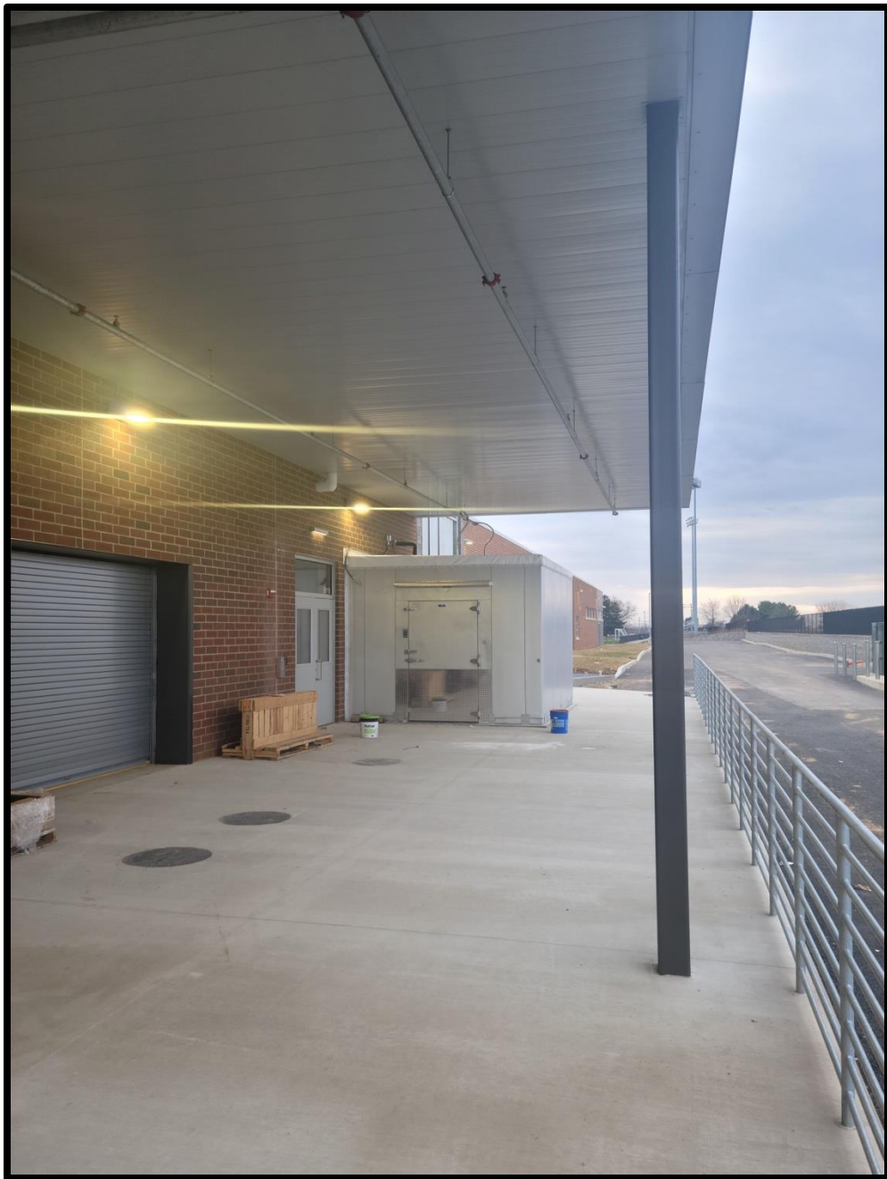
Loading Dock Walk-in Cooler
