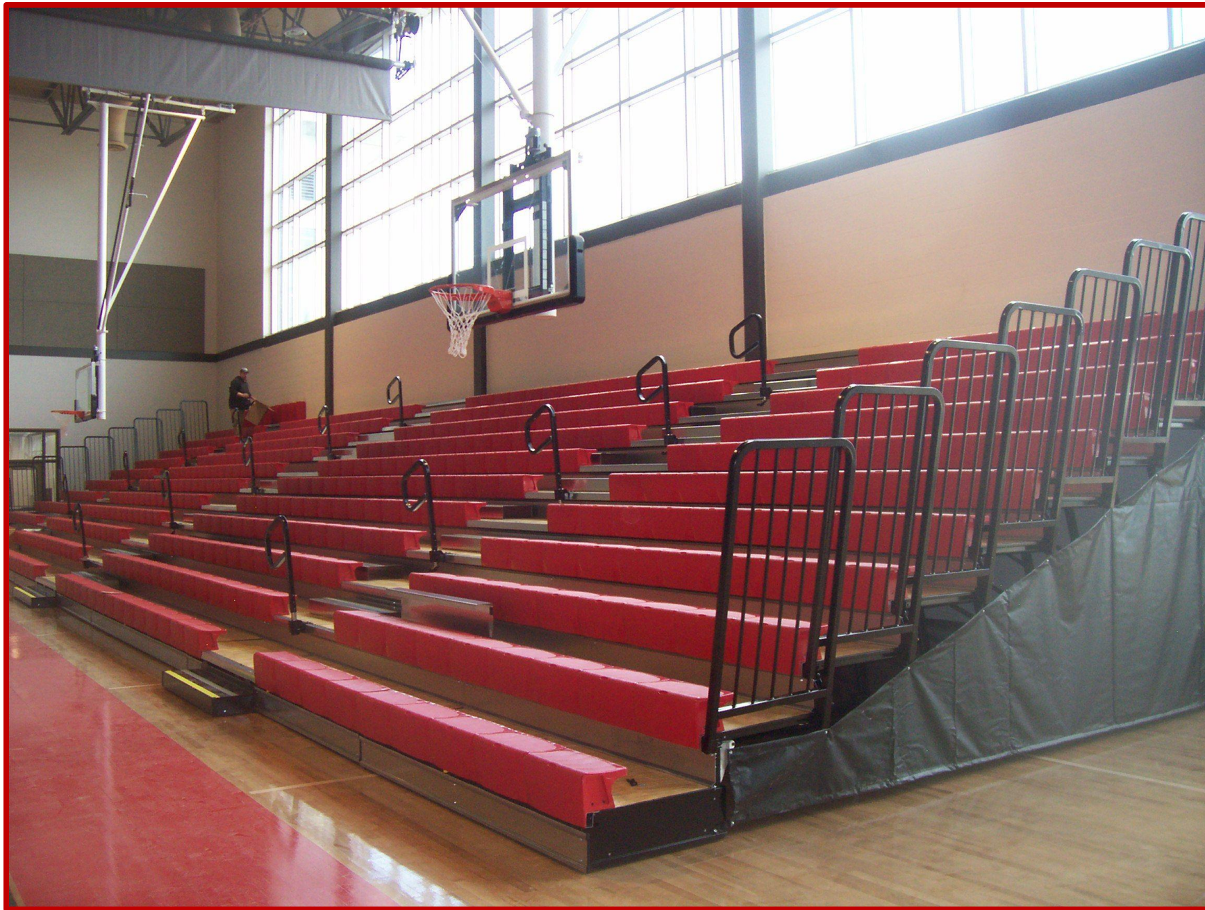
Area A Main Gym Bleachers
