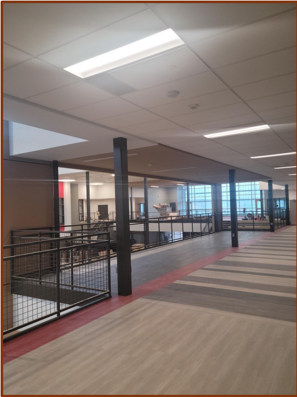
Area A – Looking at Stair E
