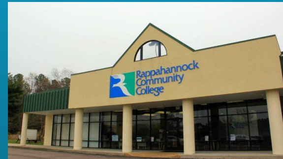
Kilmarnock Site - Workforce Center - 804-435-8970
