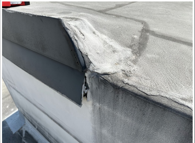
Upper Roof Flashing Sealant
