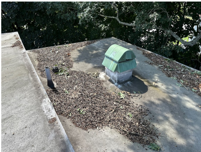
Cooper HVAC Hood Sealant
