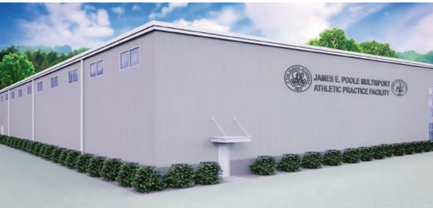
This facility will be located behind the Standish Pool and is expected to open Fall 2019.
