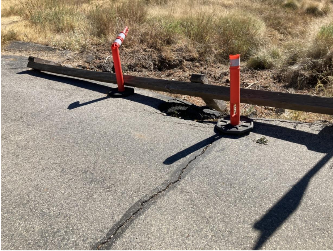
Picture # 5 - GUARD RAIL REPLACEMENT AND ASPHALT REPAIRS
