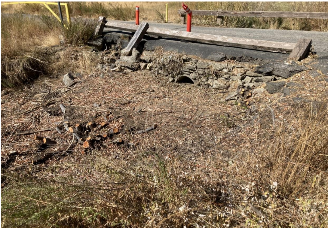
Picture #4 – GUARD RAIL REPLACEMENT AND ASPHALT REPAIRS
