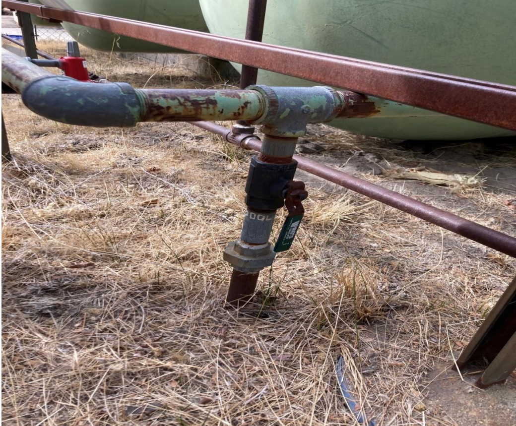
Picture #1 – Gas Valve to be cut and capped.
