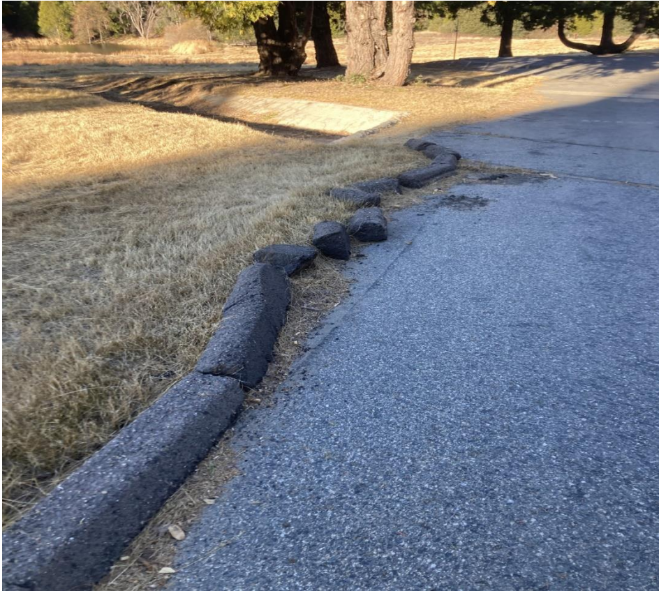
Picture #3 - ASPHALT CURB REPLACEMENT
