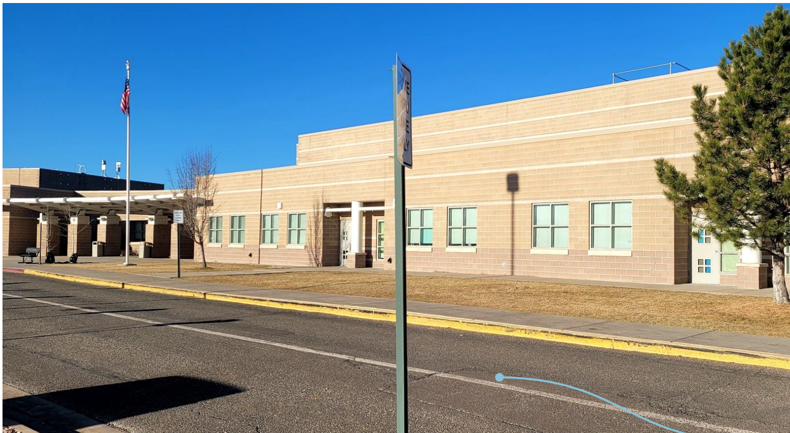
Parking Lot Asphalt Front
