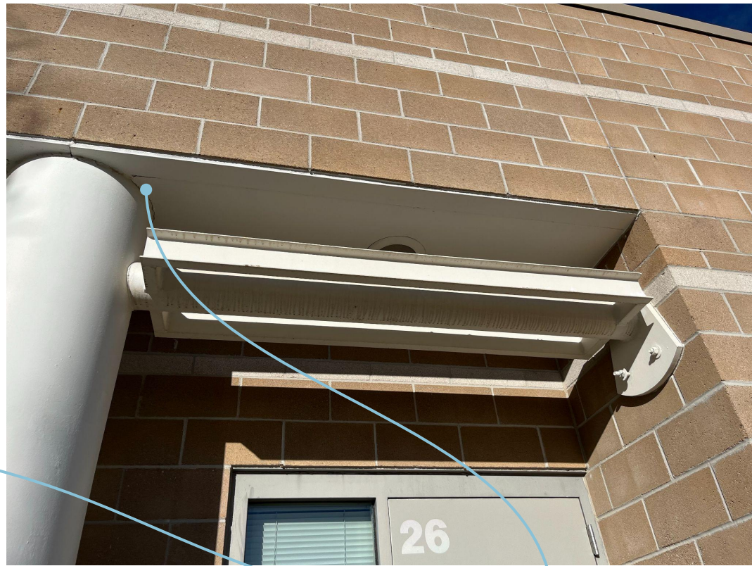
Exterior Soffits Replace gypsum with metal
