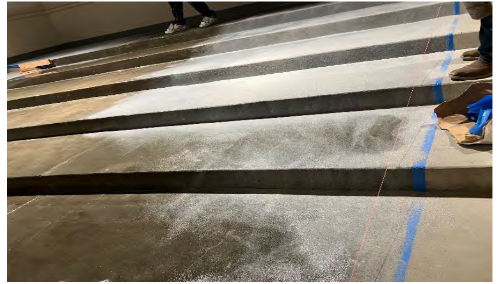
Hogan Middle School Auditorium before and after of epoxy floor installation
