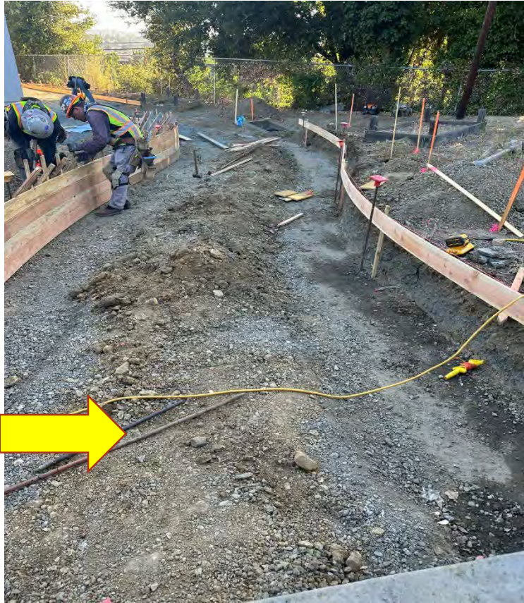
Patterson Elementary layout for new accessibility ramp located at the back of the campus
