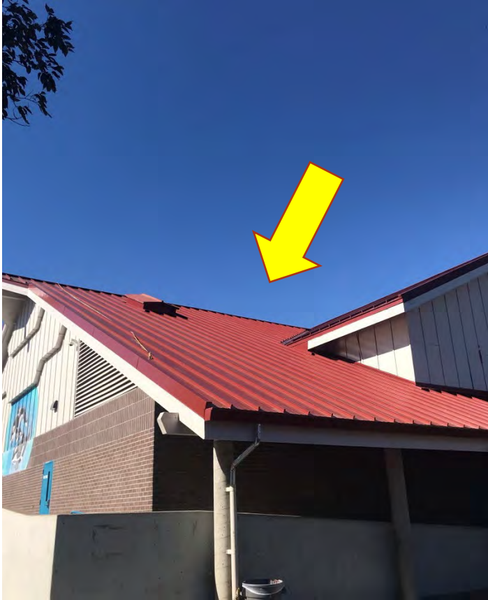
Wardlaw Elementary new roof panels installed at the Multipurpose room
