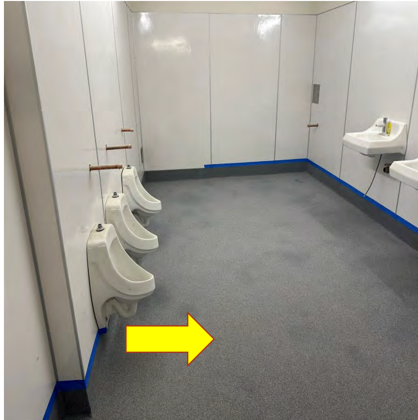
Patterson Elementary new restroom epoxy flooring
