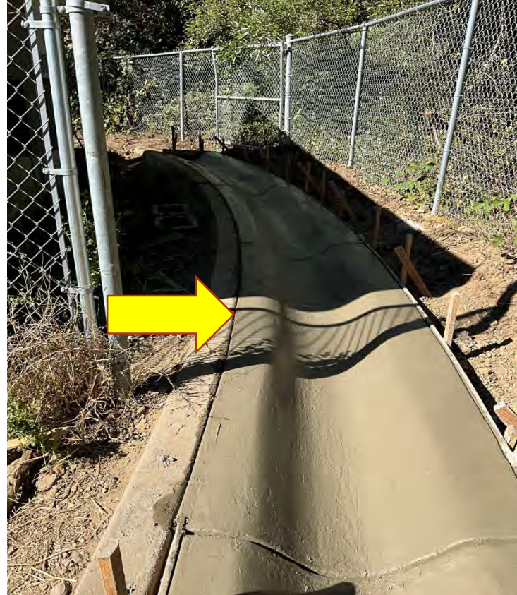
Glen Cove new v ditch for proper water flow behind the portables
