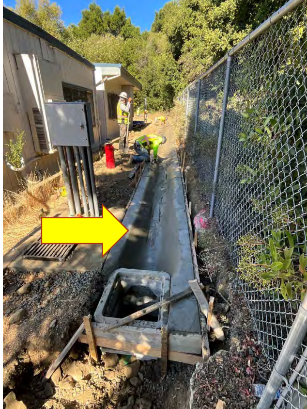
Glen Cove new v ditch for proper water flow behind the portables
