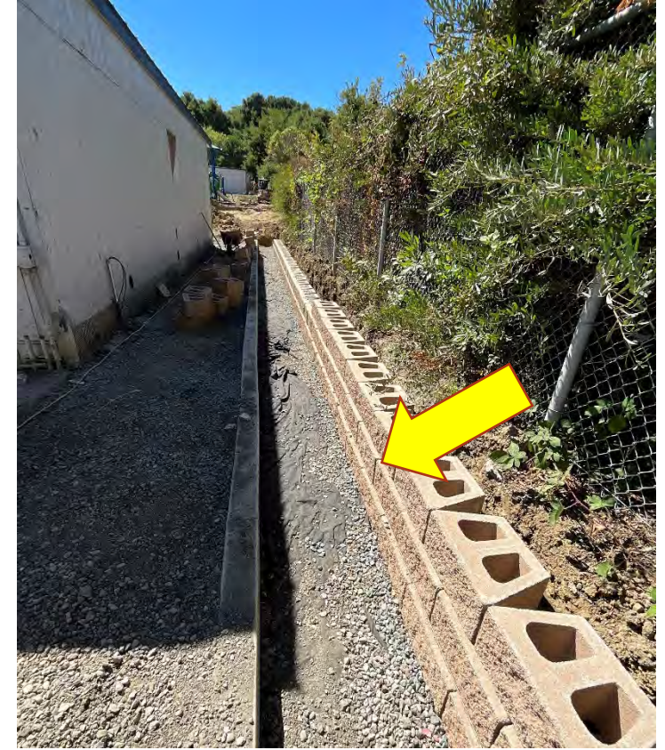
Glen Cove new French Drain for proper water flow behind portables
