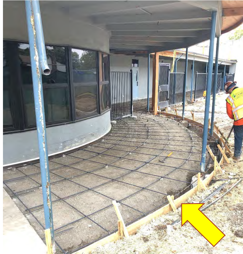
Steffan Manor Elementary concrete pour for new accessibility upgrades
