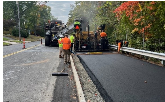
Trout Brook Trail Phase 3 Paving
