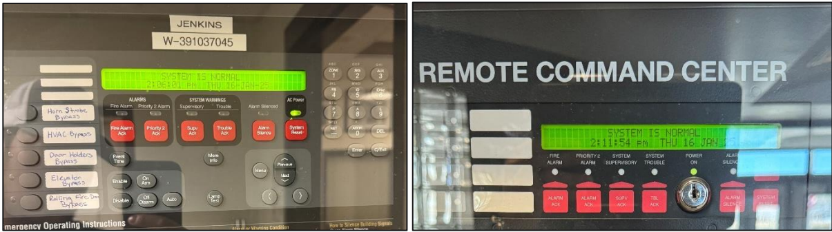
Figure 5.2. JMS Fire Alarm Control Panel and Remote Command Center
