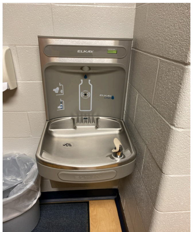
3/28/2024 - 1400-70 - Manor Hill - 002291B- Entrance to Gym
