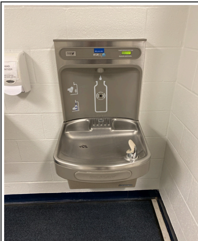
3/28/2024 - 1400-65 - Manor Hill - 001065F- Outside Gym
