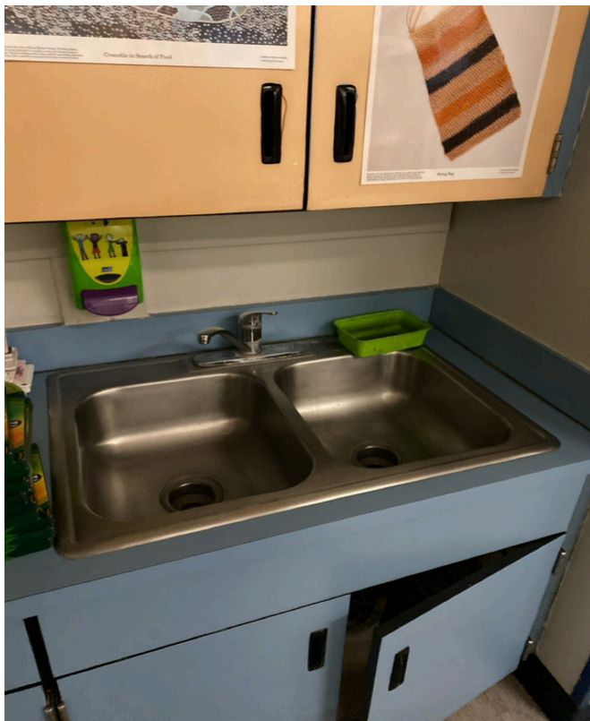
3/28/2024 - 1400-43 - Manor Hill - 001039-Room 31
