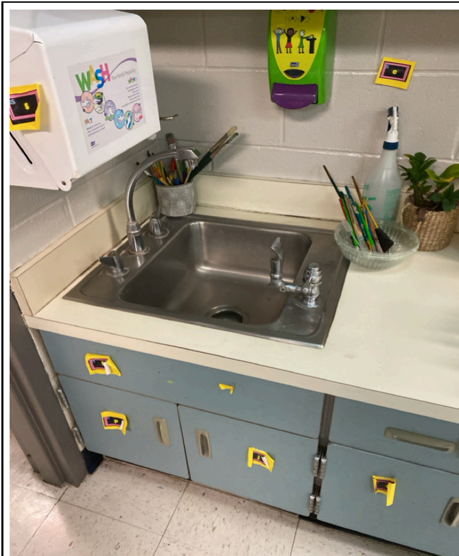
3/28/2024 - 1400-13 - Manor Hill - 002284F-Room 10
