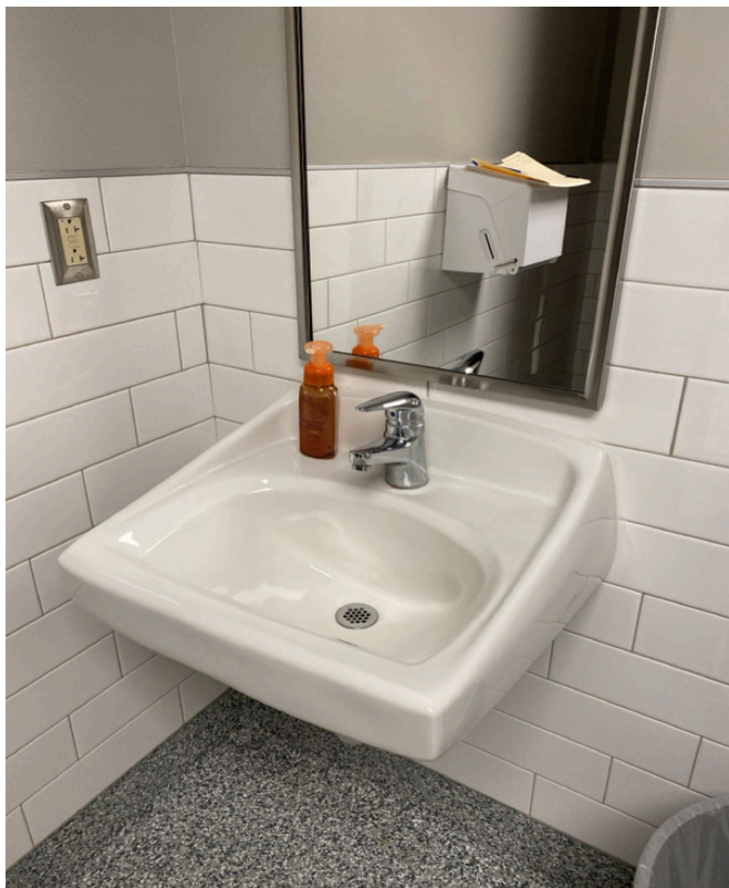
3/28/2024 - 1400-39 - Manor Hill - 002282-Staff Restroom by Nurse
