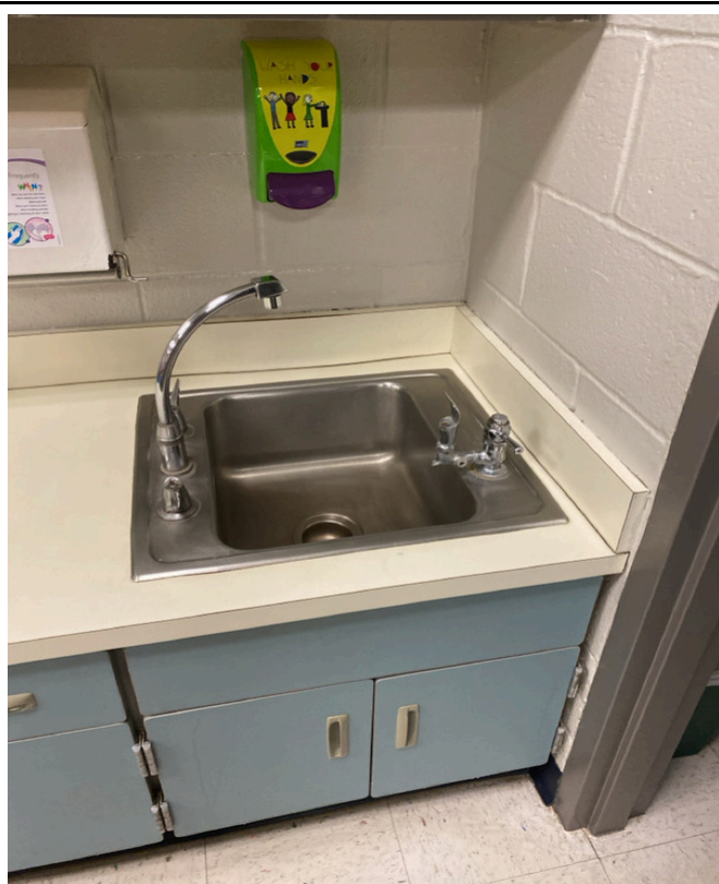
3/28/2024 - 1400-16 - Manor Hill - 001003F-Room 12
