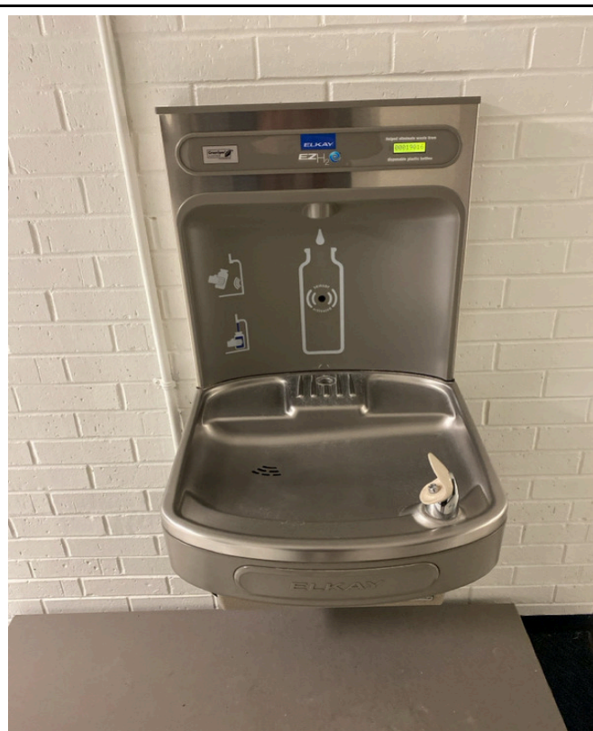
3/28/2024 - 1400-10 - Manor Hill - 001013F-By Room 11
