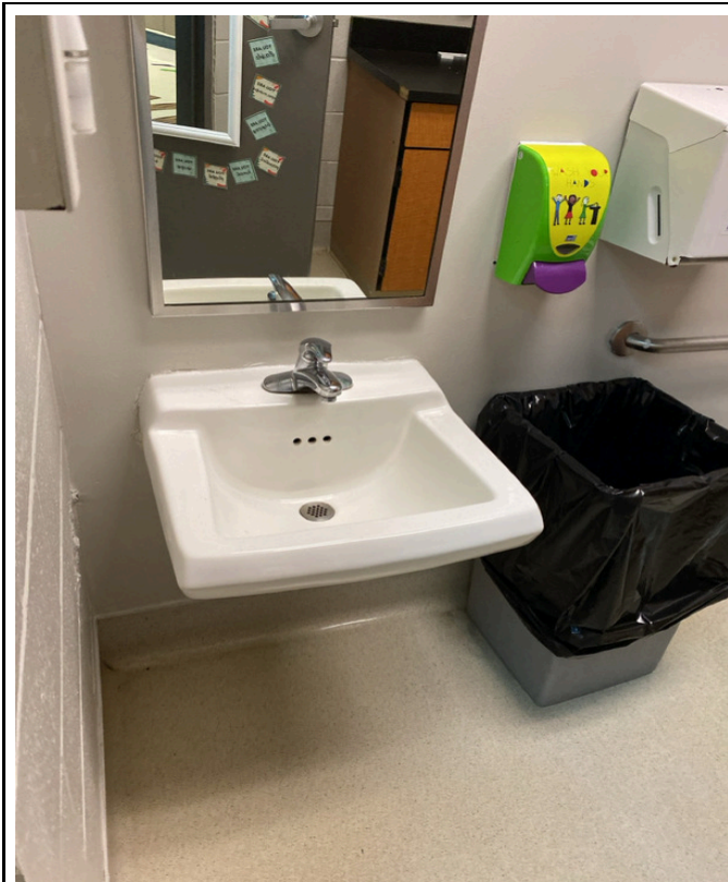
3/28/2024 - 1400-21 - Manor Hill - 001006-Room 14-Restroom
