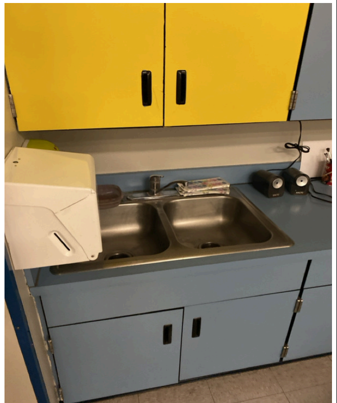
3/28/2024 - 1400-44 - Manor Hill - 001040-Room 31
