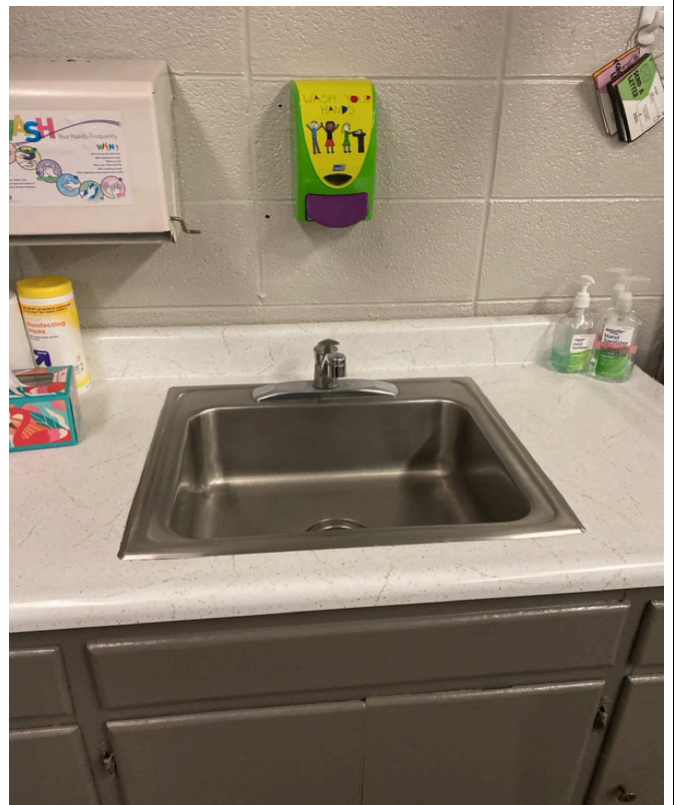
3/28/2024 - 1400-80 - Manor Hill - 001056-Room 42
