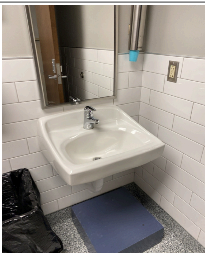
3/28/2024 - 1400-94 - Manor Hill - 002281-Nurse's Office-Restroom
