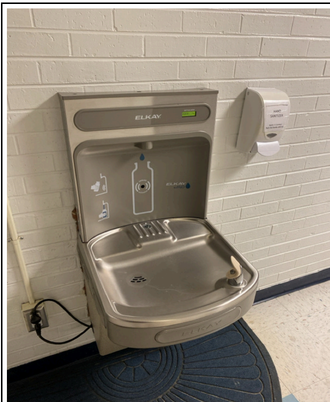
3/28/2024 - 1400-53 - Manor Hill - 002296F-By Room 35
