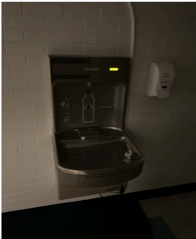
3/28/2024 - 1400-79 - Manor Hill - 001049F-By Room 44
