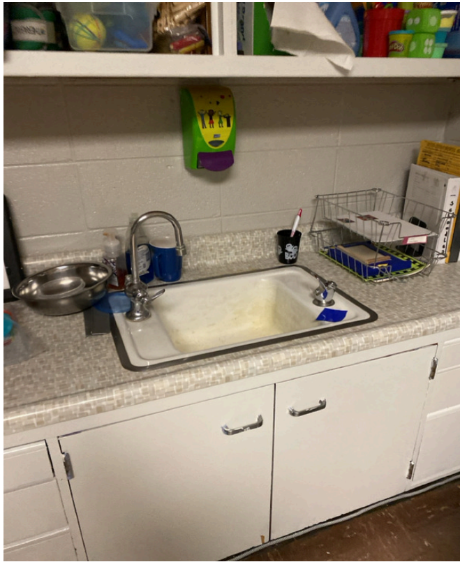
3/28/2024 - 1400-37 - Manor Hill - 001033F-Room 15A
