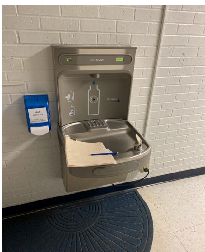
3/28/2024 - 1400-30 - Manor Hill - 002283F-By Room 13
