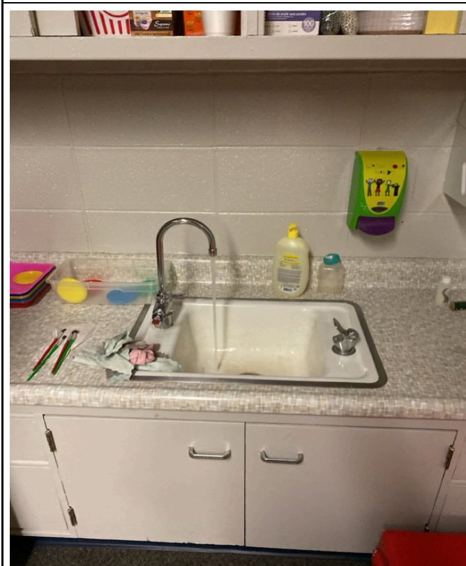
3/28/2024 - 1400-11 - Manor Hill - 001015-Room 11
