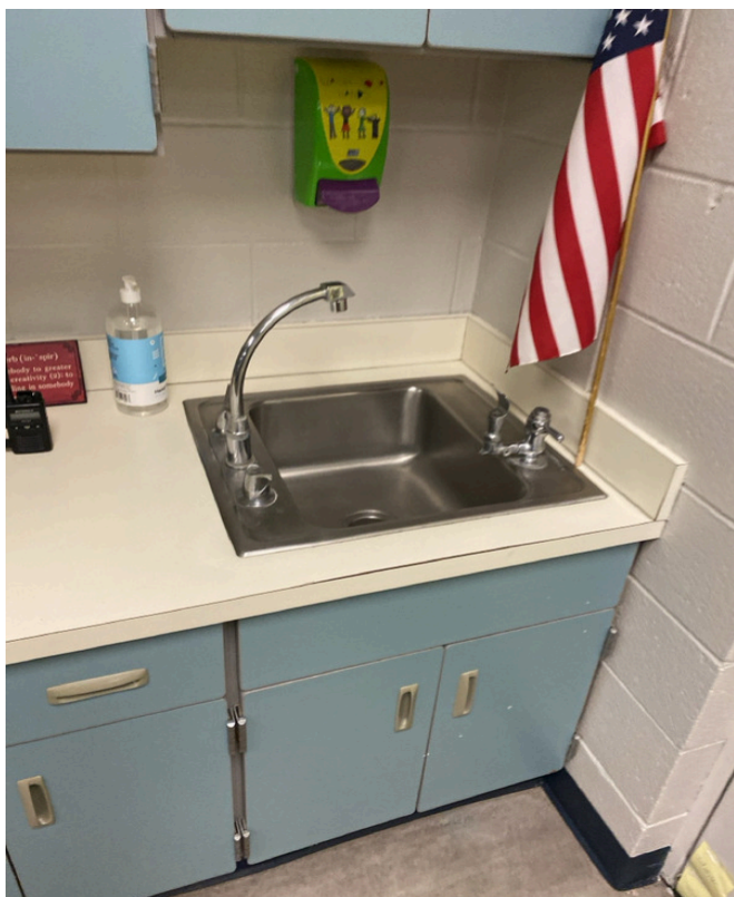
3/28/2024 - 1400-19 - Manor Hill - 001005F-Room 14
