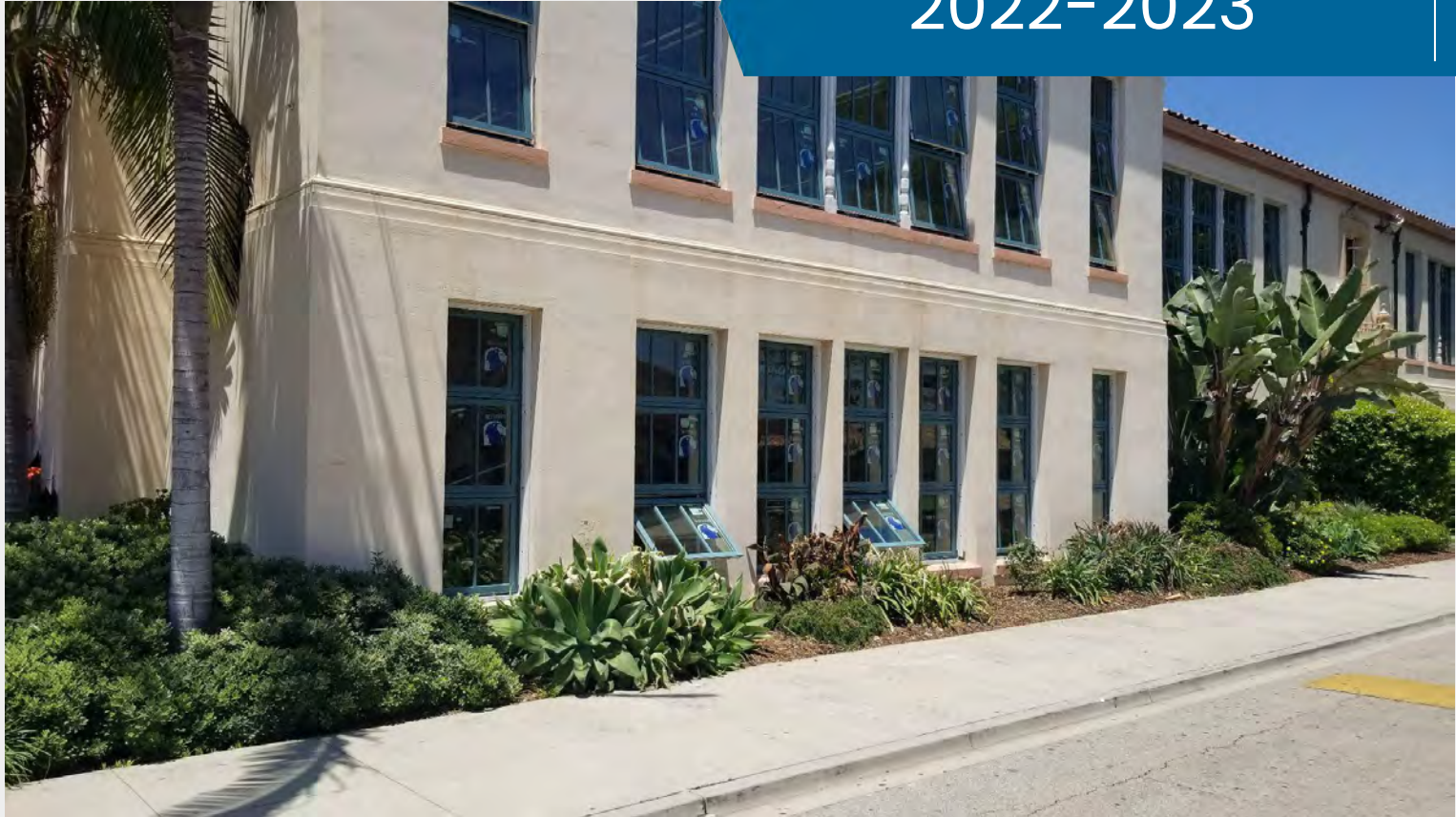
SBHS Windows Rehabilitation (In progress)
