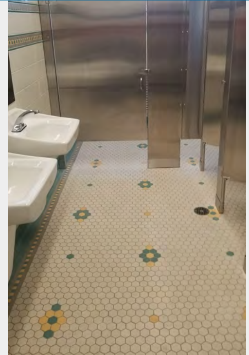
SBJHS Restrooms Upgrades
