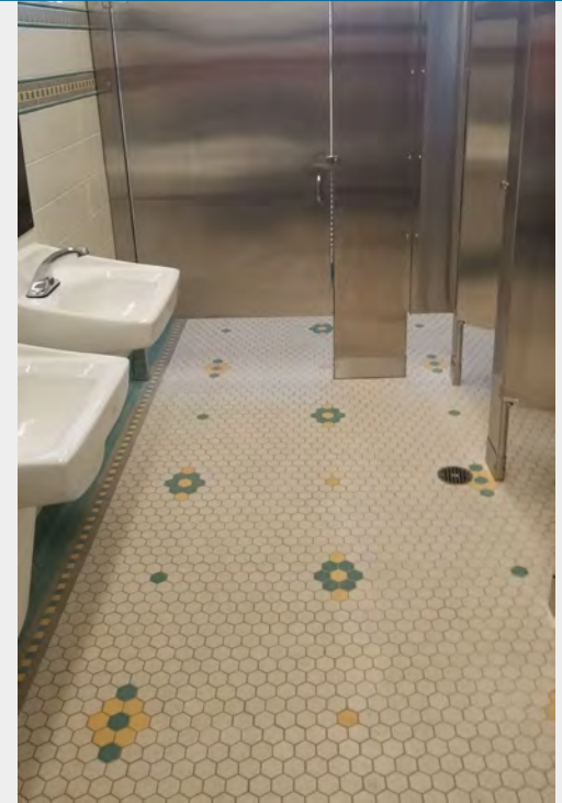
SBJHS Restrooms Upgrades
