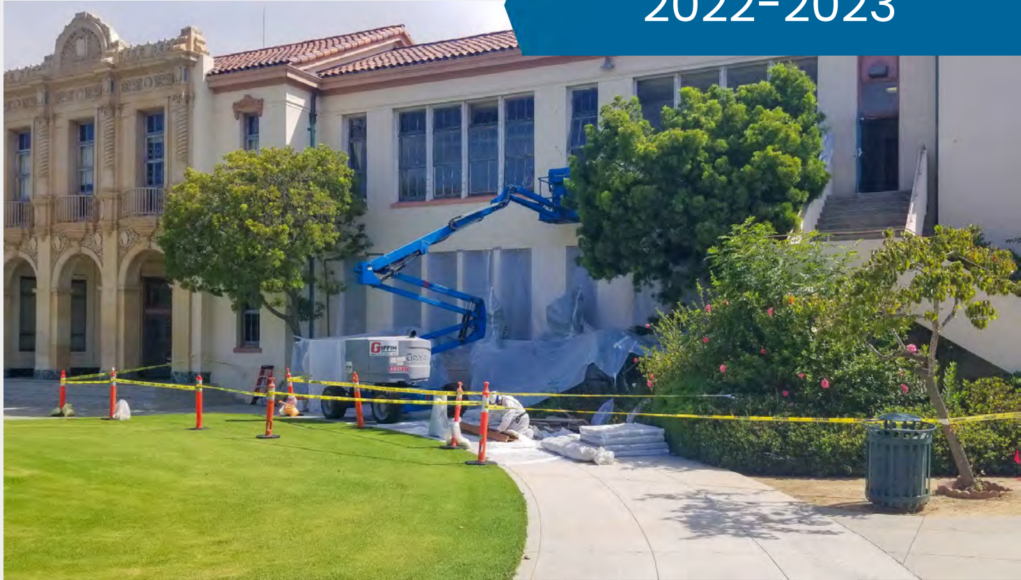
SBHS Windows Rehabilitation (In progress)
