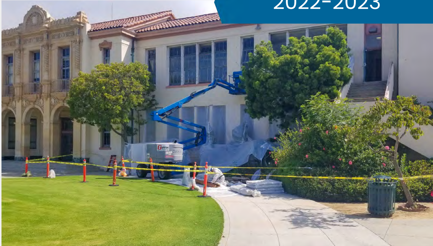
SBHS Windows Rehabilitation (In progress)
