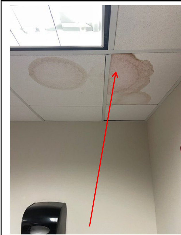
Photo 1: View of Room C119 with stained ceiling tiles. No visible mold growth present.
