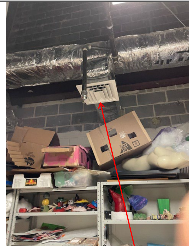
Photo 7: View of A173 Storage room. Ceiling level supply diffuser recently cleaned.
