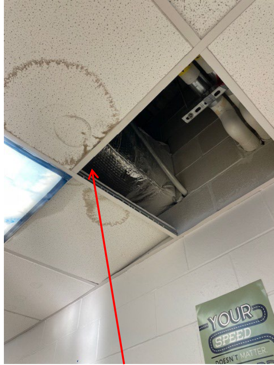
Photo 2: View of missing/stained ceiling tiles in Room A173 below pipe chase.
