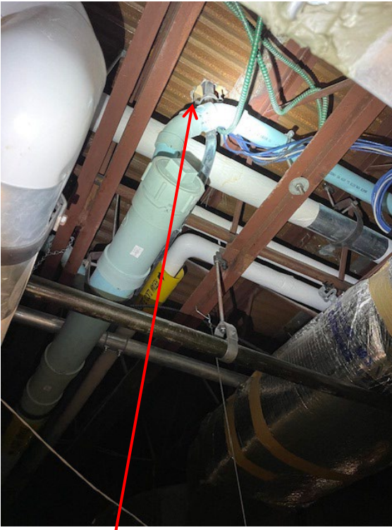
Photo 1: View of Room A173 ceiling plenum above stained tiles. Opening in steel decking above water and drain piping may allow for condensation dripping.
