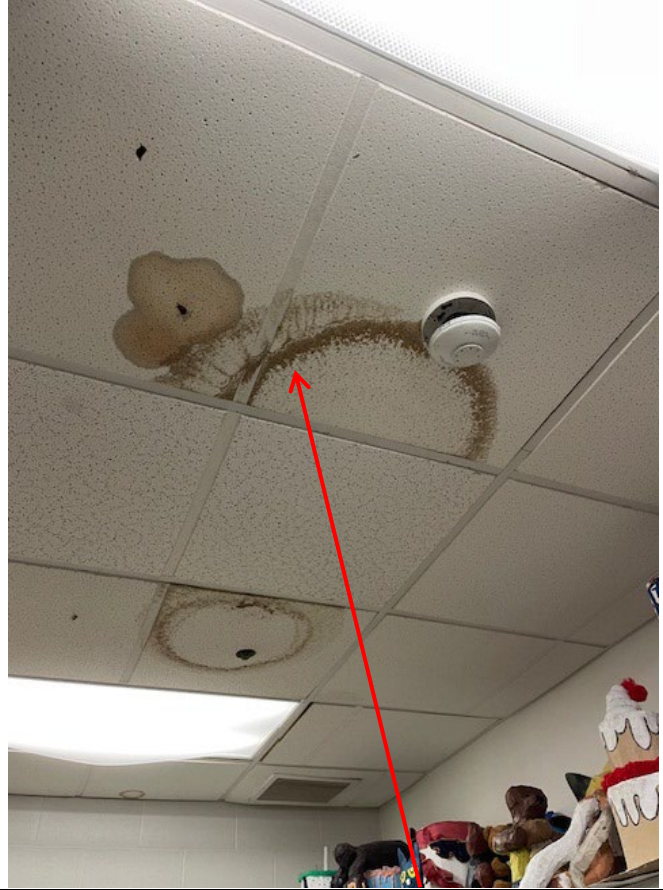
Photo 6: View of Art Room middle Kiln Room: Stained ceiling tiles present. Investigate plenum above and replace tiles.
