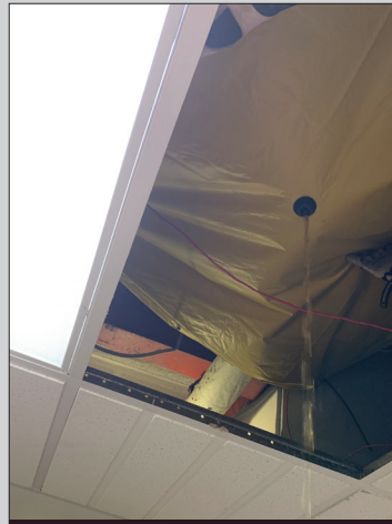
Active Water Leaks
