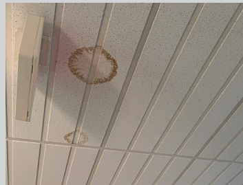
Stained and Water Damaged Ceiling Tiles
