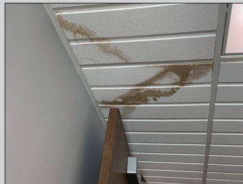
Stained and Water Damaged Ceiling Tiles
