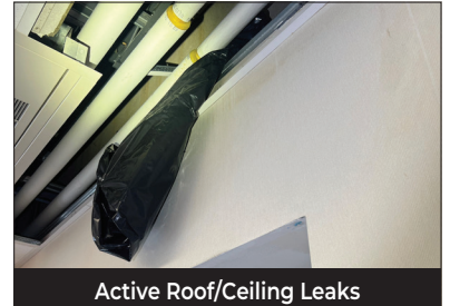
Active Roof/Ceiling Leaks
