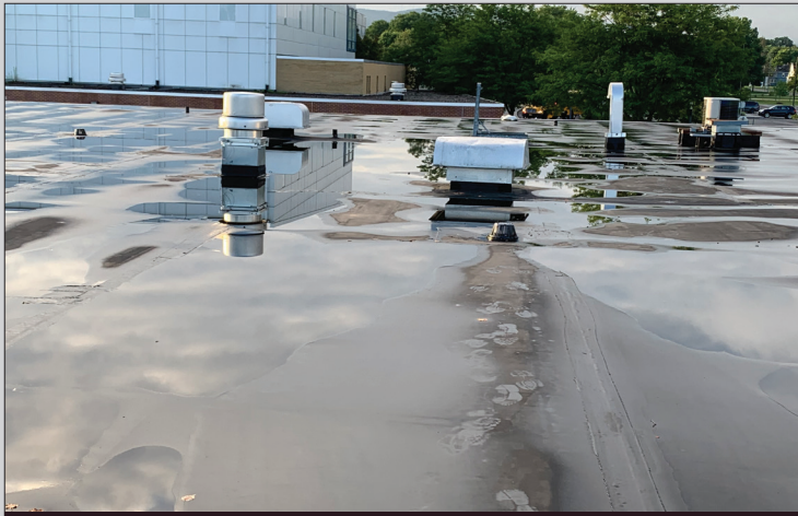
Water Pooling on Primary School Roof
