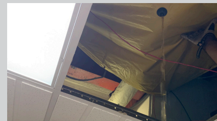
Active Roof/Ceiling Leaks
