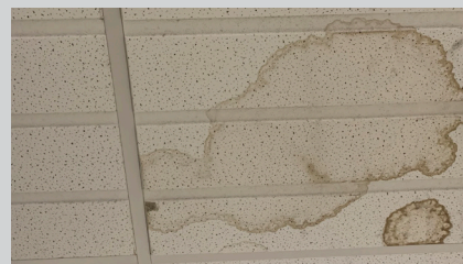
Stained/Damaged Ceiling Tiles
