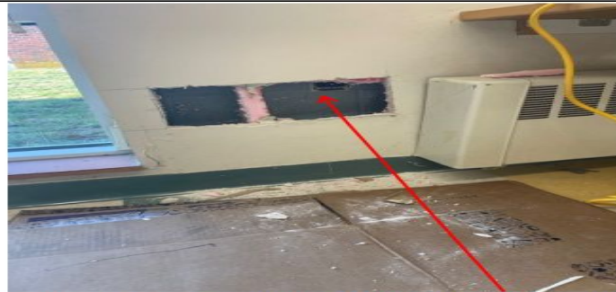
Photo 3: View of classroom 140 at perimeter wall. No suspect mold growth within wall cavity. Original block wall outlet allows outside air leakage to enter wall cavity.
