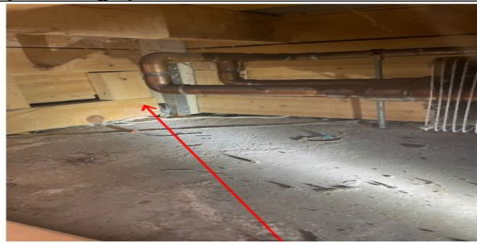
Photo 2: View of Classroom 240 under perimeter bench top at heat piping/radiation unit with bare concrete floor. Wood support joists dry with no visible mold. Suspect mold growth on underside of bench top (not pictured).
