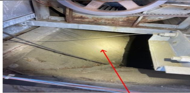
Photo 4: View of ACU1 servicing library. Accumulated dirt and suspect mold growth on damaged/frayed interior duct liner at vertical supply duct.
