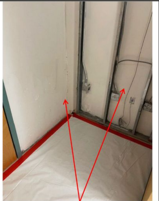
Photo 2: View of 203 closet front right corner showing wallboard removed and back side of exposed wallboard encapsulated. Remaining surfaces decontaminated.
