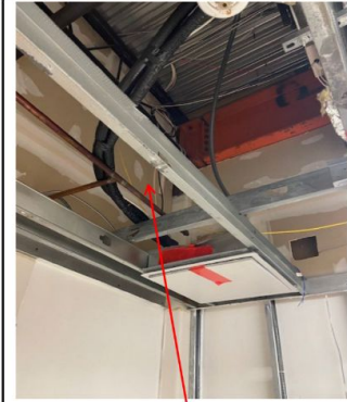
Photo 3: View of room 203 closet into ceiling plenum. Ceiling board and moldy pipe insulation removed and surfaces decontaminated.
