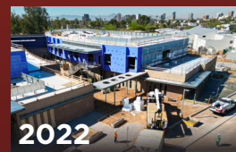
Madison Park Middle School Construction
