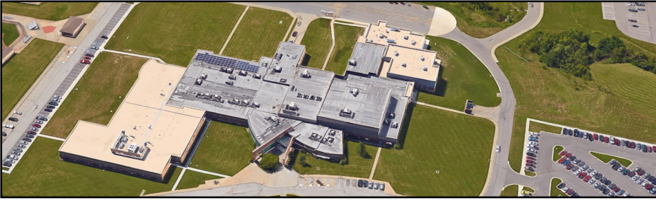
Figure 166. Aerial view of Belton High School.
