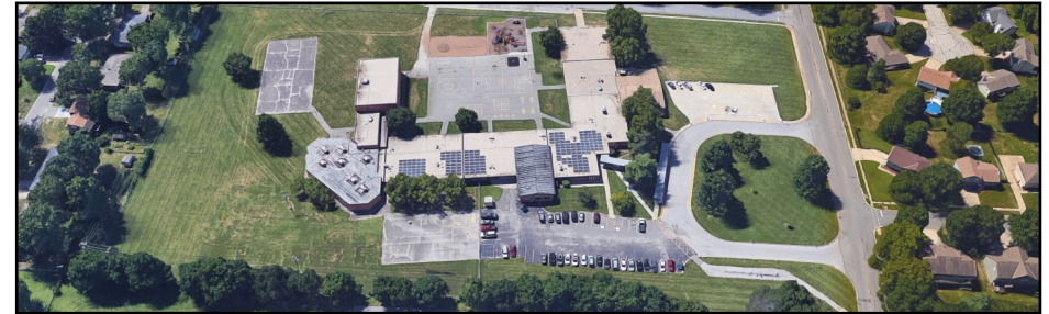
Figure 142. Aerial view of Gladden Elementary School.
