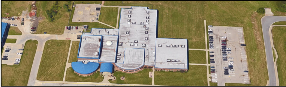
Figure 156. Aerial view of Mill Creek Elementary School.
