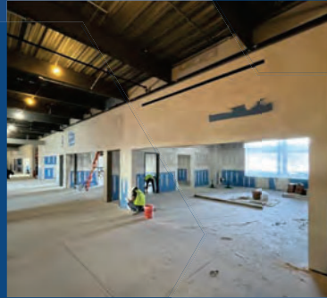
First Floor Drywall Finishing
