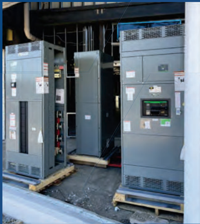
Main Distribution Panel Install
