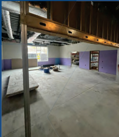
First Floor Drywall Install
