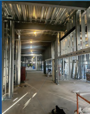
First Floor Interior Framing
