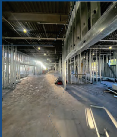
Second Floor Interior Framing
