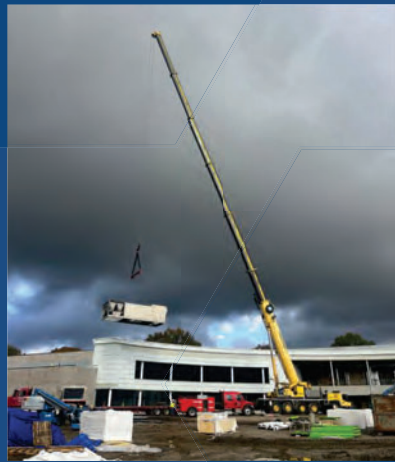
RTU Installation
