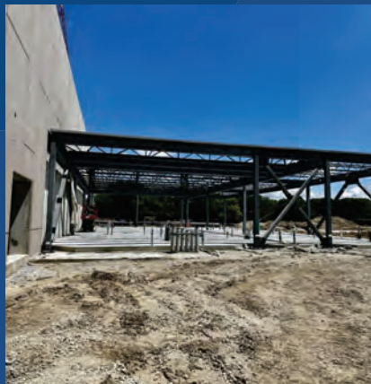
Kitchen Structural Steel Erection
