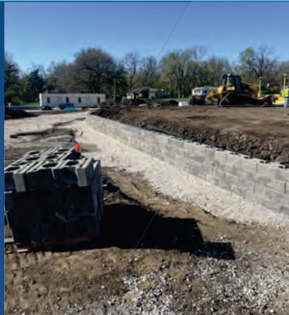
Retaining Wall Install
