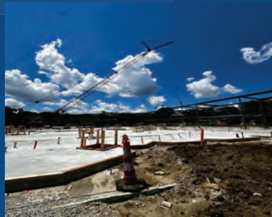
Completed Concrete Slab
