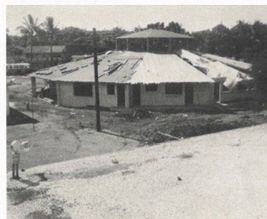
We are not outdoors any longer. We have a roof now.
