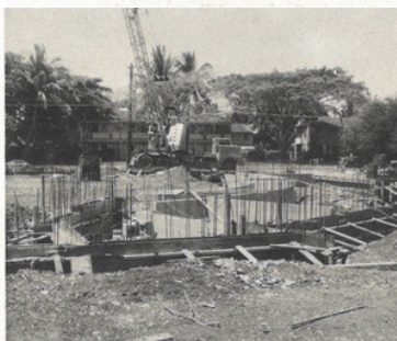
Remember the big hole with all the supports and steel rods?
