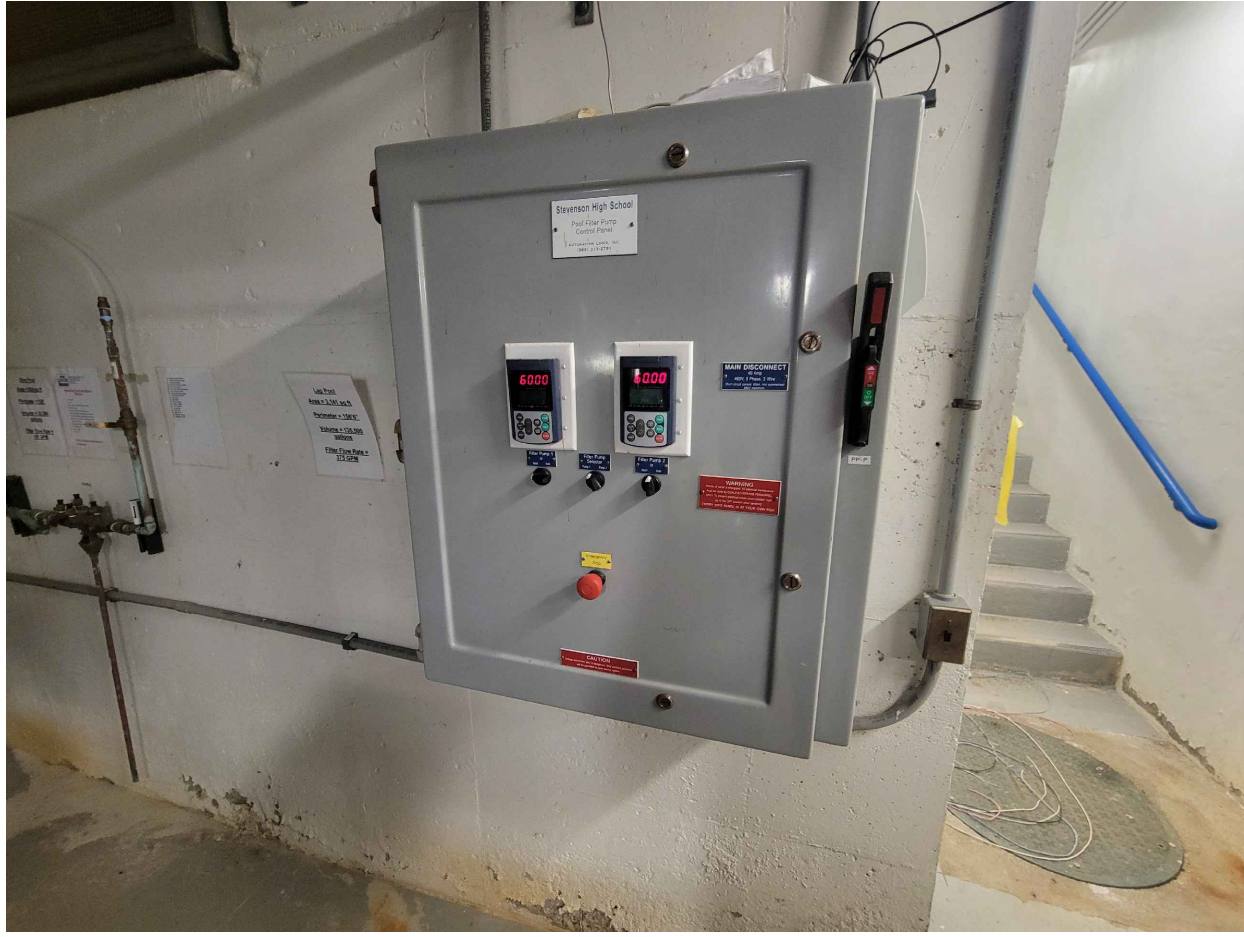
5 AQ0.3 EXISTING PUMP MOTOR STARTER NTS
