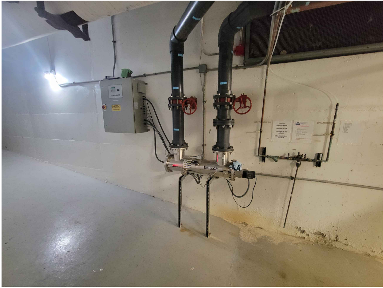
8 AQ0.3 EXISTING UV CHAMBER & CABINET NTS
