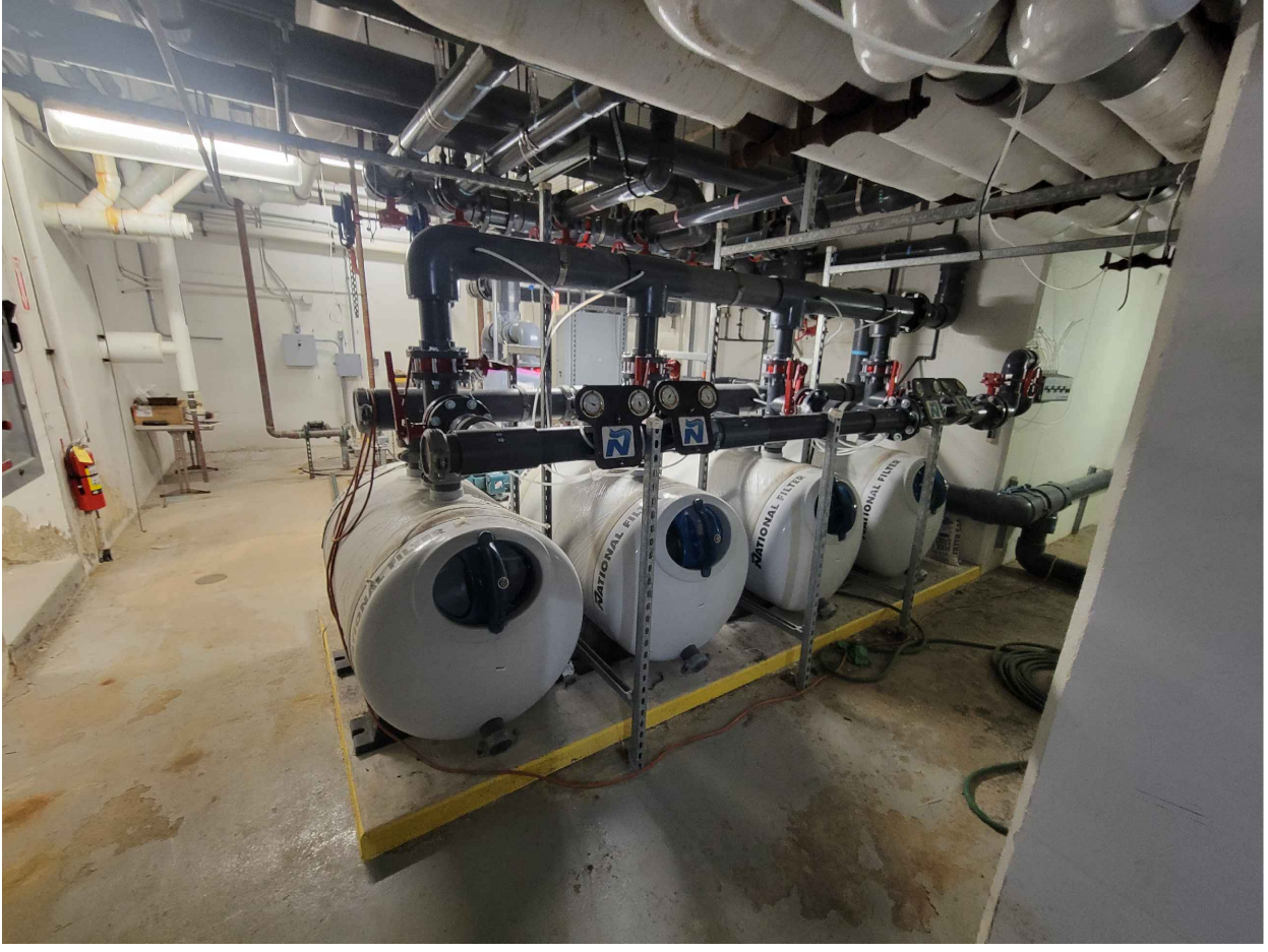
4 AQ0.3 EXISTING SAND FILTERS NTS
