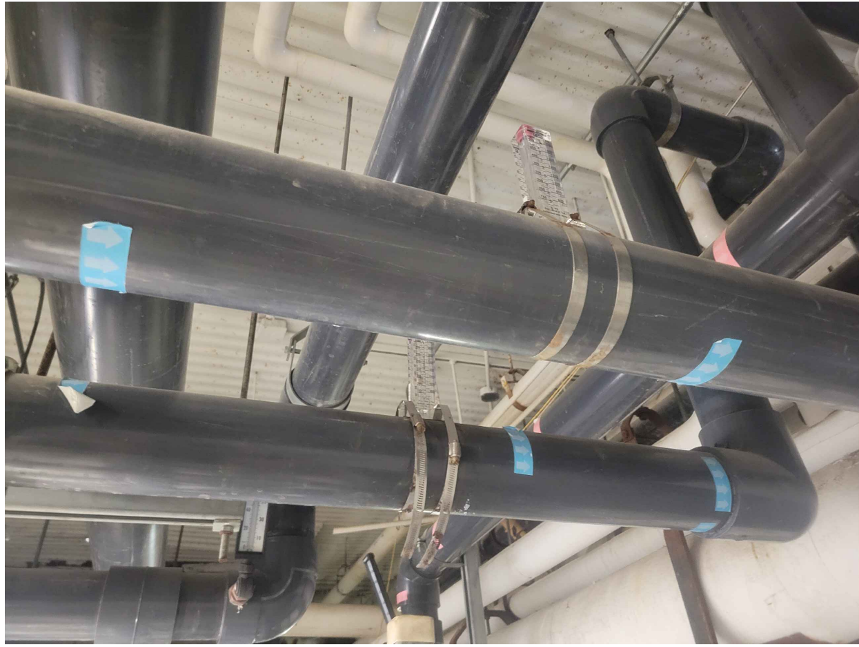
7 AQ0.3 EXISTING FLOW METER SENSORS NTS
