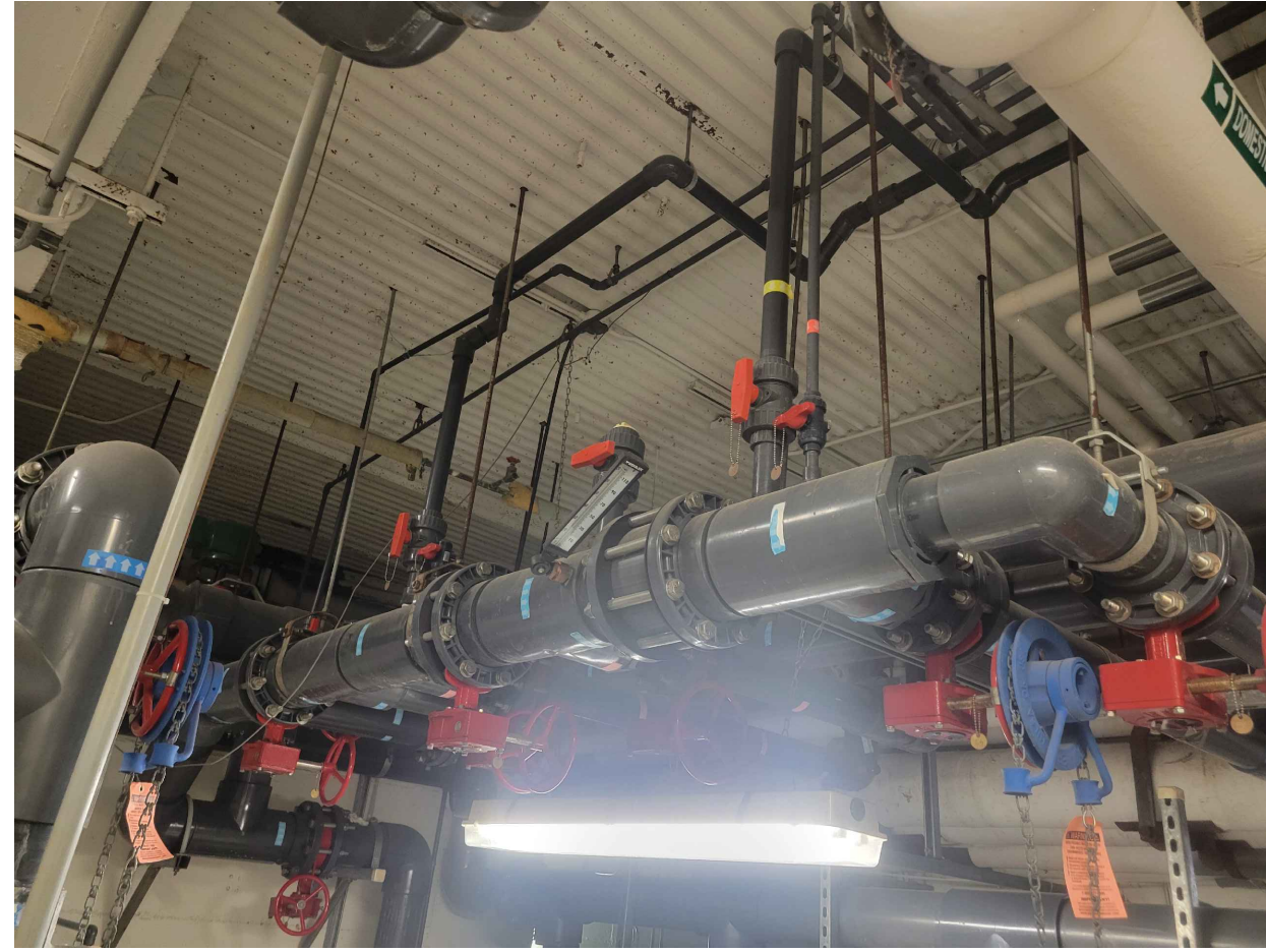
11 AQ0.3 EXISTING CHEMICAL INJECTIONS NTS
