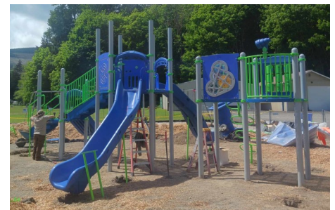
New playground equipment construction in progress.
