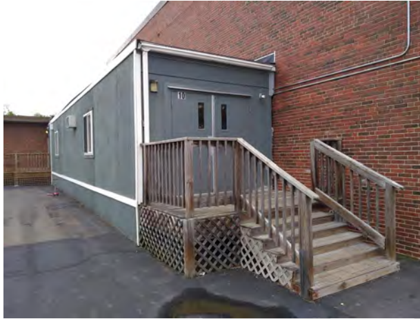
8. Modular addition has deteriorated and leaks at connection to main building.
