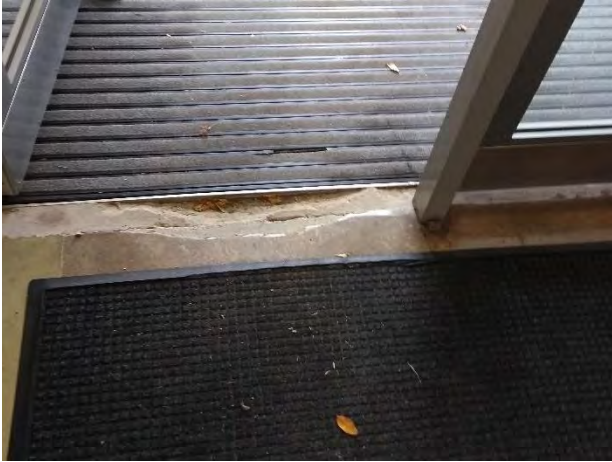
7. Threshold at entry is damaged. Walk off matt is worn.
