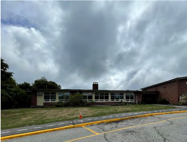
1. Bituminous driveway shows signs of cracking and freeze/thaw damage.
