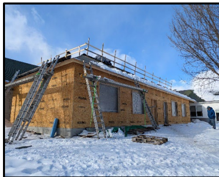
New classrooms on the backside of the building!
