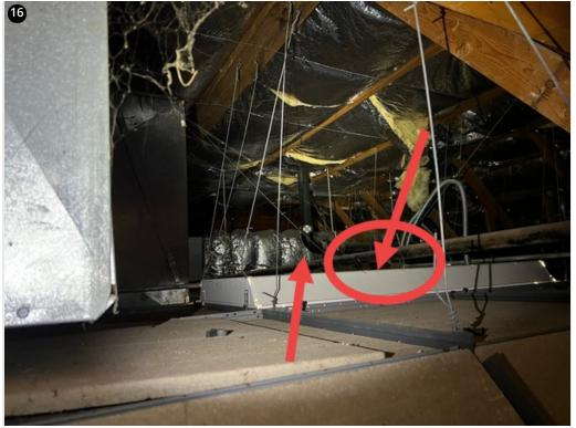
This is either the middle west or the southwest drain, leaking has been reported in this area although the tiles that had water stains were about 5 feet closer to where I am standing, not directly below the drain.
