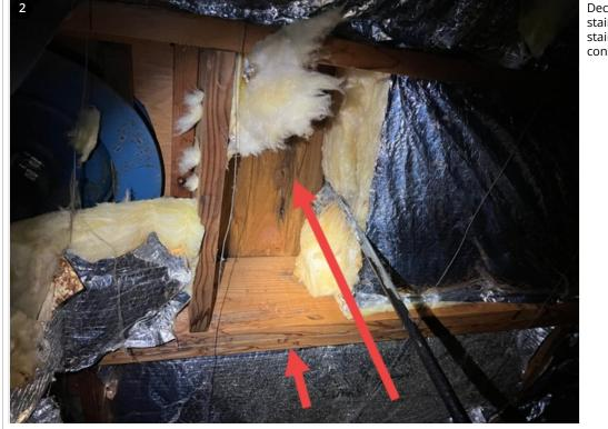
Decking shows the majority of the water staining and dry-rot. All areas of water staining on the structural members did not consist of dry rot, of what we could see.
