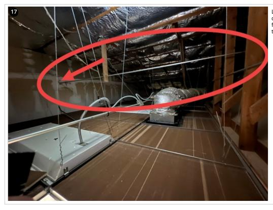
Leaks in the past have caused major drywall damage and repairs noted to have come from water following this conduit pipe down through the other side of the wall.
