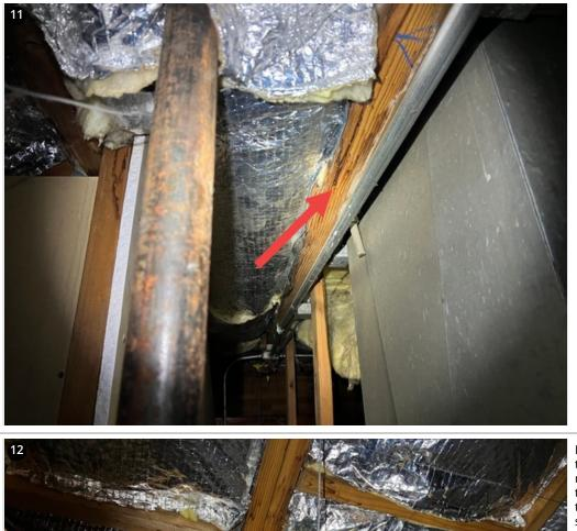
In the photos it is hard to tell, but many of the areas on the wood that look to have moisture are simply just sap coming out of the wood. During my inspection I was able to identify these because the light on the sap produced a shiny effect whereas the water staining would not.
