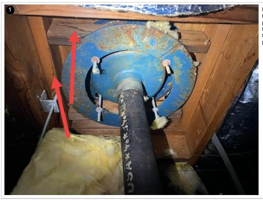
East side drain, minor water staining around the drain. This drain had been a leak problem many times but not often coming through the roof or top of the drain, most of the time it was coming from the connection point farther down the drain pipe.
