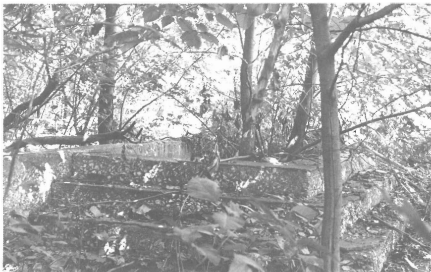
Huge trees grow inside the foundation today. Finish concrete has eroded away from risers of the steps.
