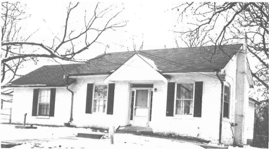
Photo taken in March, 1969, shows addition built to the west wall by present owners, Salem Baptist Church. West chimney is gone, east chimney is relocated, gable is now above entry. Cistern cap at left is all that remains of well.
