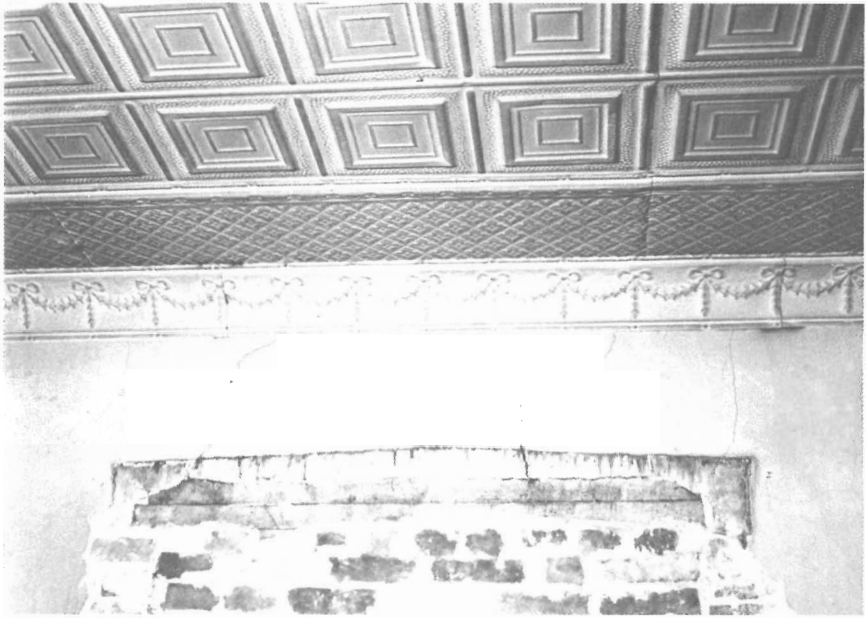
The Koders bricked up the top part of the old, high windows, and installed a lower ceiling. This is the view in the attic today. The window lintels and tin ceiling serve to date the building in the 1870s or 1880s.
