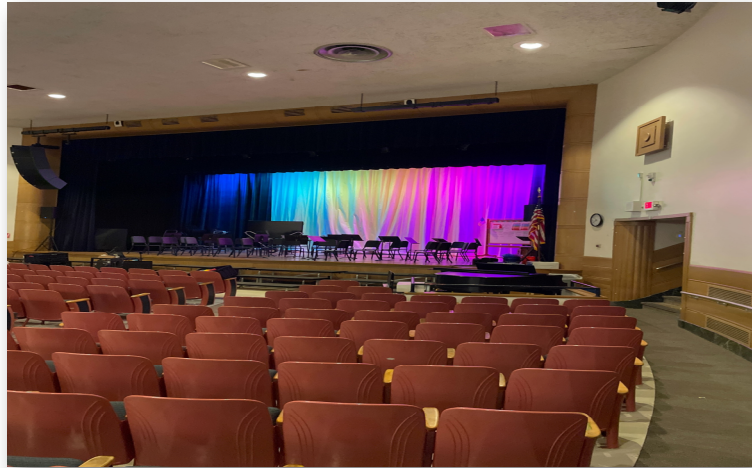
WBS - Testing of lighting during owner training
