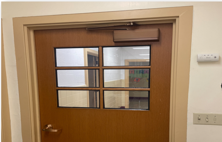
WBS - Door hardware replacement
