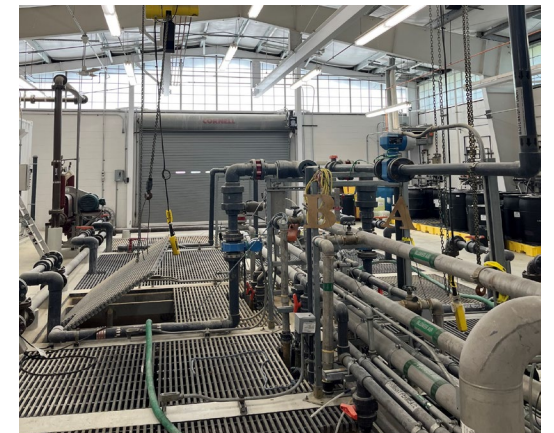
WASTEWATER TREATMENT FACILITY (2009)
