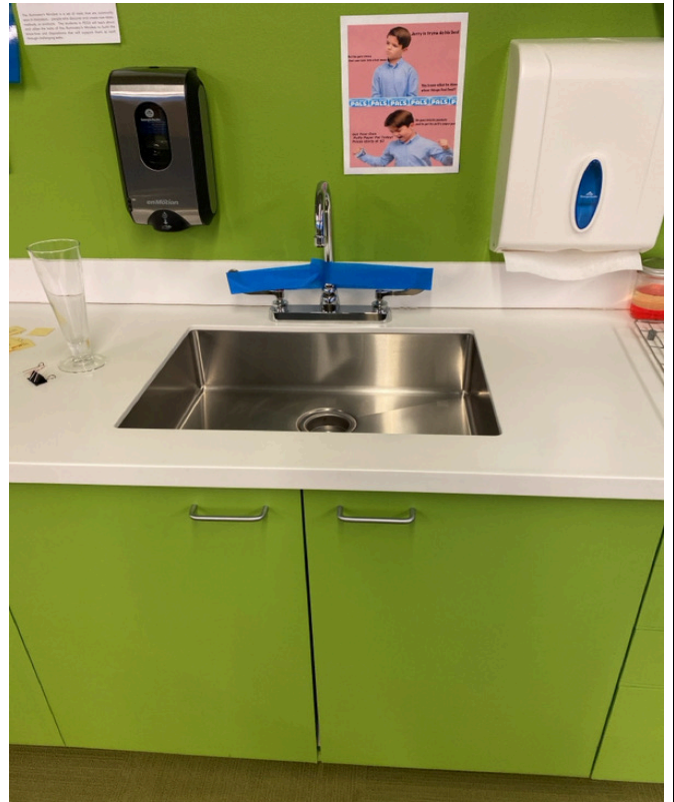
1/31/2025 - 6889-18 - NIC - 1st Floor Northwest Sink
